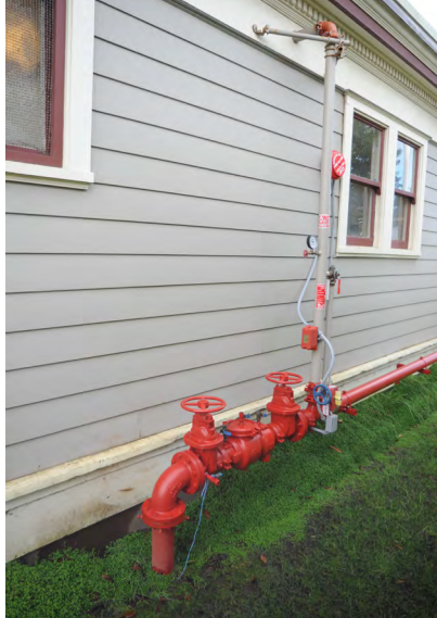
FIRE SPRINKLER RISER SERVING CITY HALL EAST
