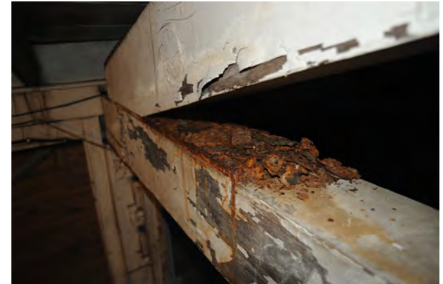
HEAVILY CORRODED POOL TRUSS HEEL CONNECTION IN SOUTH WING LOW BAY SPACE
