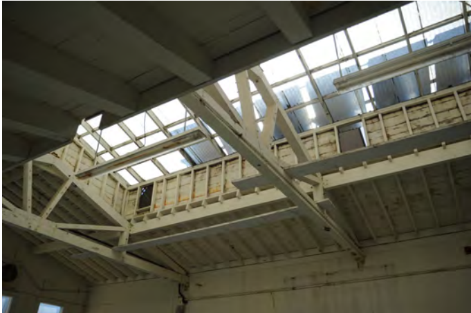
ATRIUM AND WOOD TRUSSES IN POOL BUILDING
