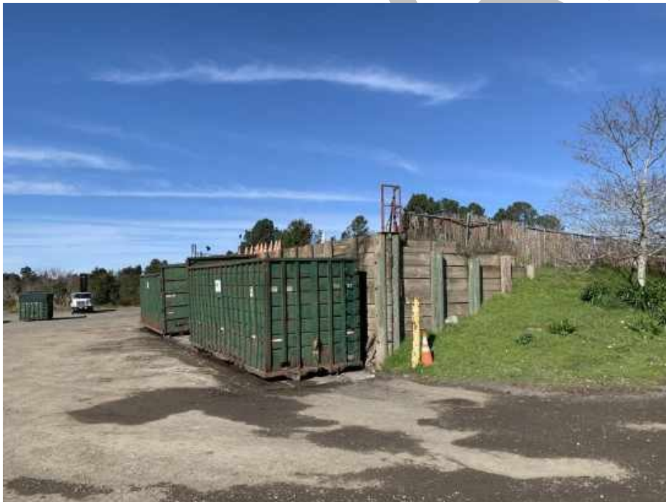
Photo 6: Current Z-wall for Load-out into Debris Boxes
