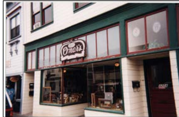
Transom windows are important elements of original storefronts and should be restored when possible
