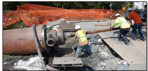
SHN supervised the force main installation under Pine Hill.
