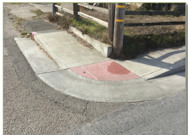
Woodward Street - Non compliant ADA ramp, need to edge grind so AC does not build up at lip of ramp
