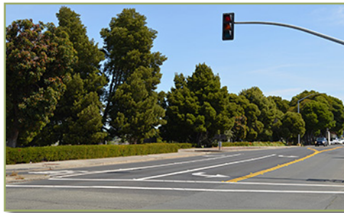
Superelevated Roadway Transition Into the New Mare Island Bridge Western Approach (Above).
