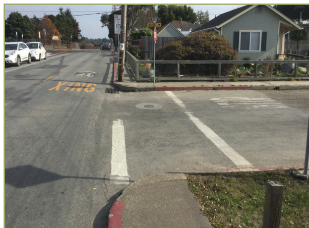
Olsen Lane - Utility covers to raise to grade, conform grades at intersection
