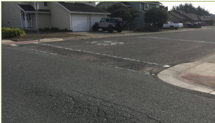
Espey Way - Dig-outs, potential for concrete valley gutter
