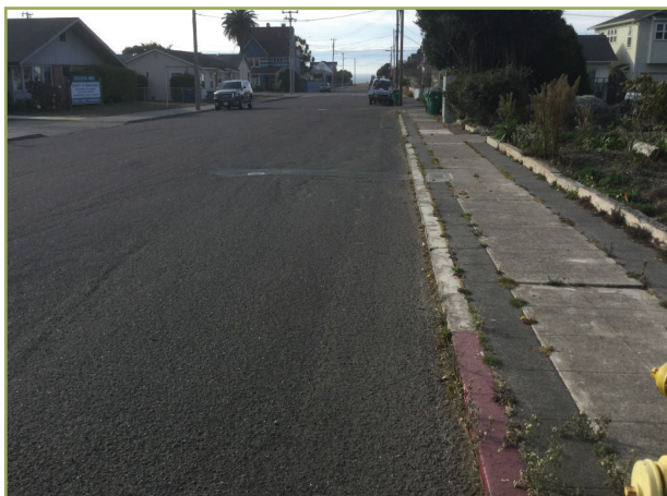
Fir Street - Need to edge grind at curb, watch cross-slopes
