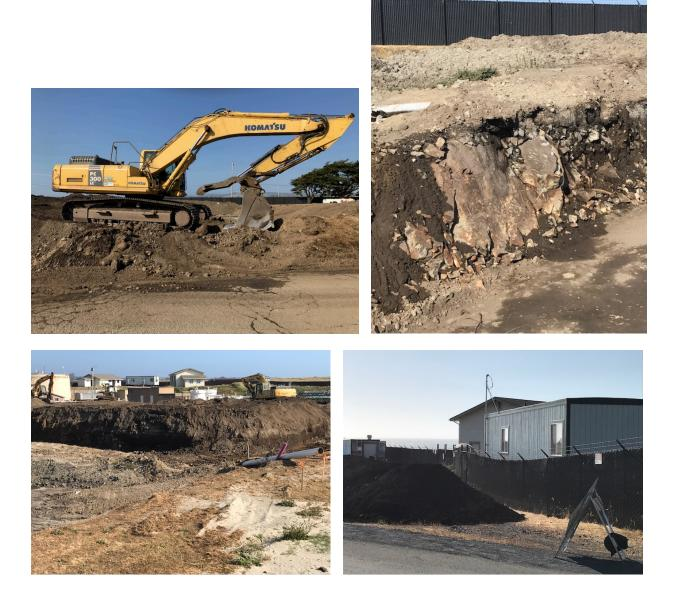
**Two Week Look Ahead** The excavation for the biological treatment tank will continue. Material from the excavation is currently being stockpiled south of the plant on City property for reuse. Topsoil will be utilized to create a grassy berm around the southerly and easterly fence lines of the WWTP, while denser rockier material will either be placed in a permitted location near the stockpiles or used as backfill for the project.
