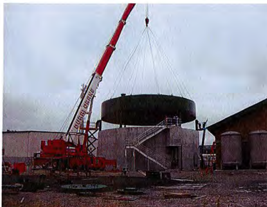
Installation of floating cover for anaerobic digester.
