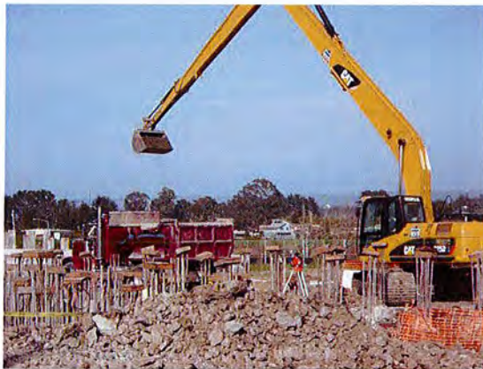
Long reach excavation, backfill and grading.
