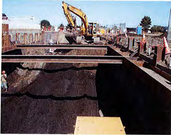
MBR Building and Tank Excavation at Crescent City WPCF.
