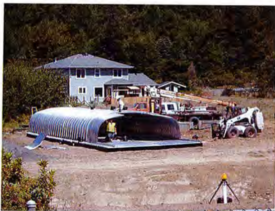
Assembly of arch culvert (Phase 1).
