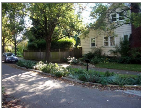
An example of a curb extension with a stormwater planter in Portland, Oregon.
