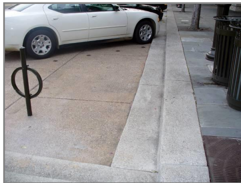
A "two-step" curb that links the parking lane and sidewalk.
