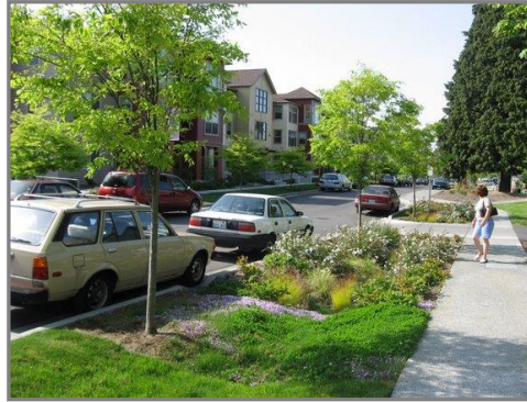
Swales are linear depressions adjacent to the streetscape that can detain and convey stormwater along their length.
