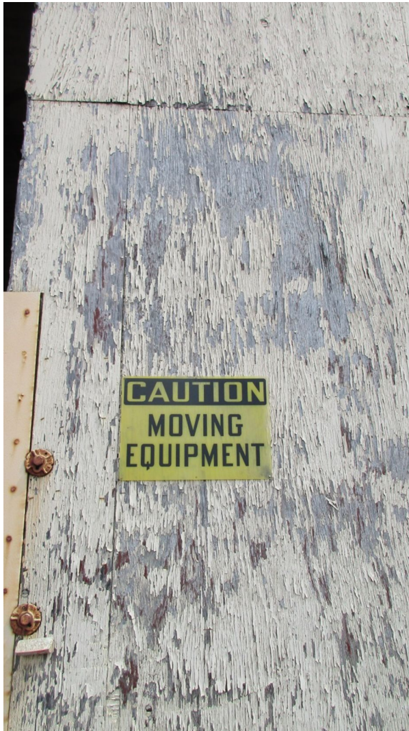
Typical deteriorated paint on external walls
