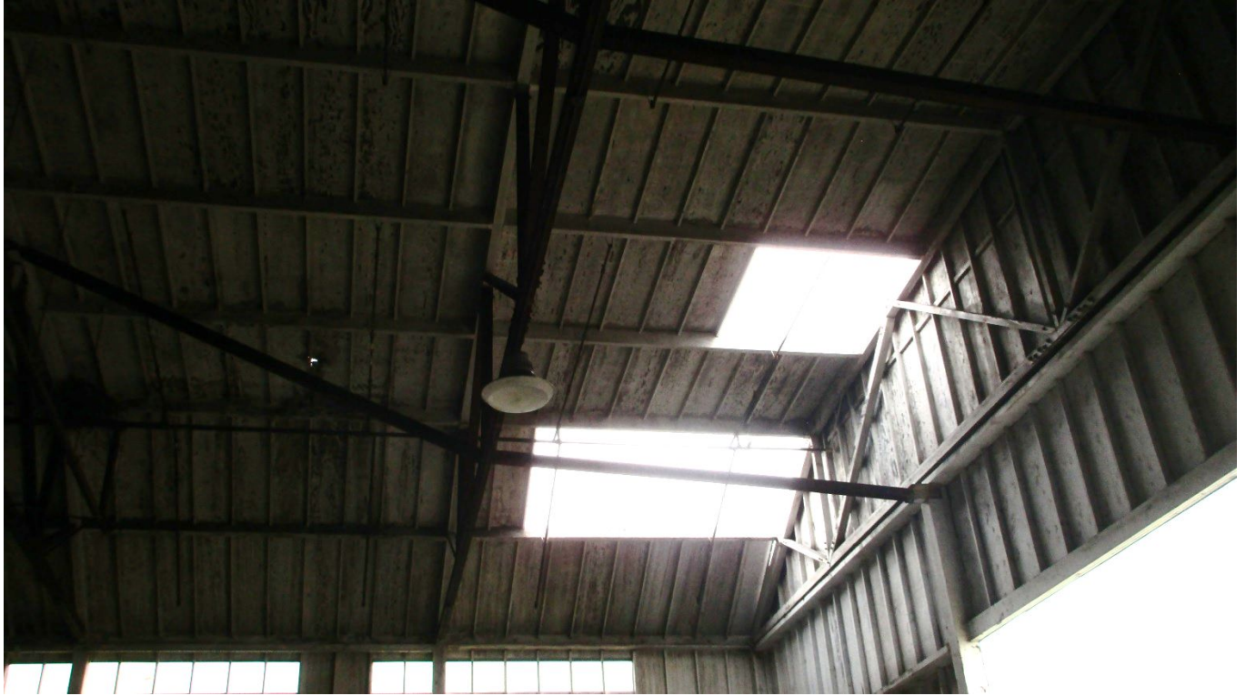
Hole in roof, interior shot
