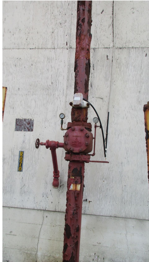
Deteriorated sprinkler main
