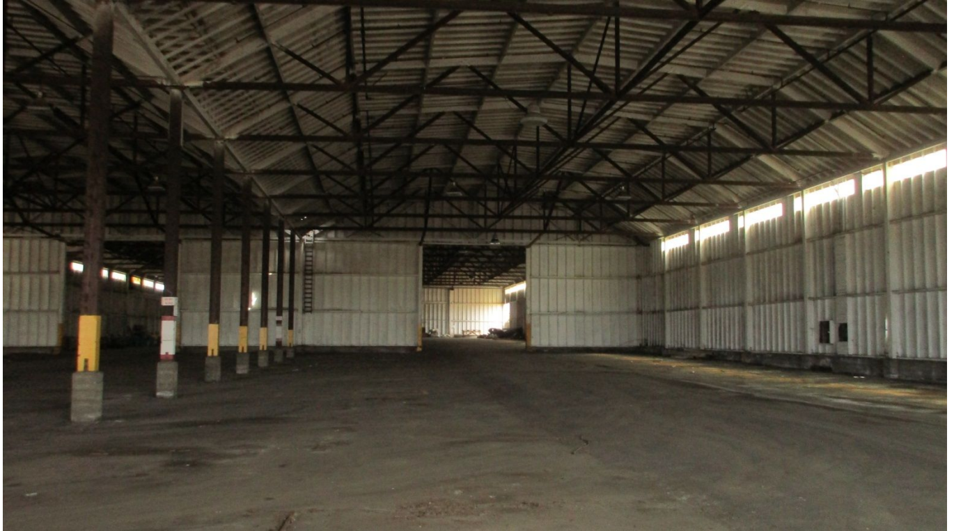
South east bay looking north, illustrates wall framing/CMU, roof structural system and asphalt floors
