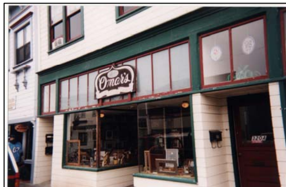
Transom windows are important elements of original storefronts and should be restored when possible
