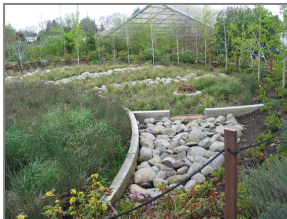
Rain gardens are landscaped planters that are more extensive than storm water planters and typically are designed to infiltrate storm water. They can be located in or adjacent to the street.
