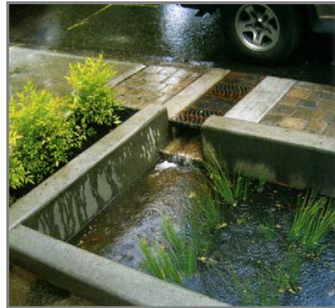
Stormwater planters allow roadway runoff to flow into and out of adjacent landscaping, where the stormwater is detained and treated.
