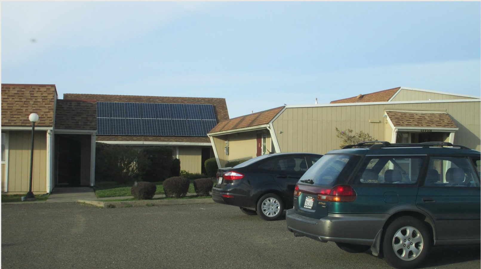
21 KW Roof Mount Solar Array
