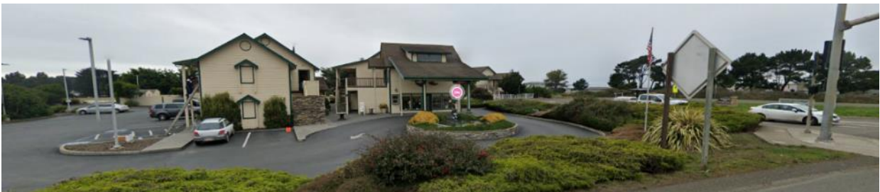
Image 1: Emerald Dolphin Motel Building A (right) and Building B (left)
