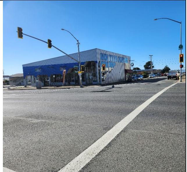
Image 6: Standard Galvanized Pole Intersection
