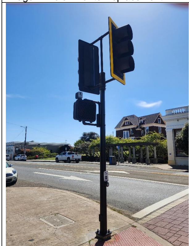
Image 3: Pole after replacement and Paint
