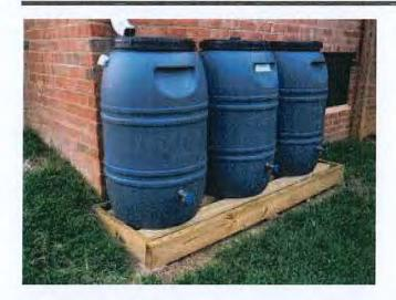
Rain Barrels and Cisterns are a system that collects and stores stormwater runoff from a roof or other impervious surface. These typically have overflow mechanisms or plugs that drain to a vegetated area or to the storm drain system when the barrel is full.
