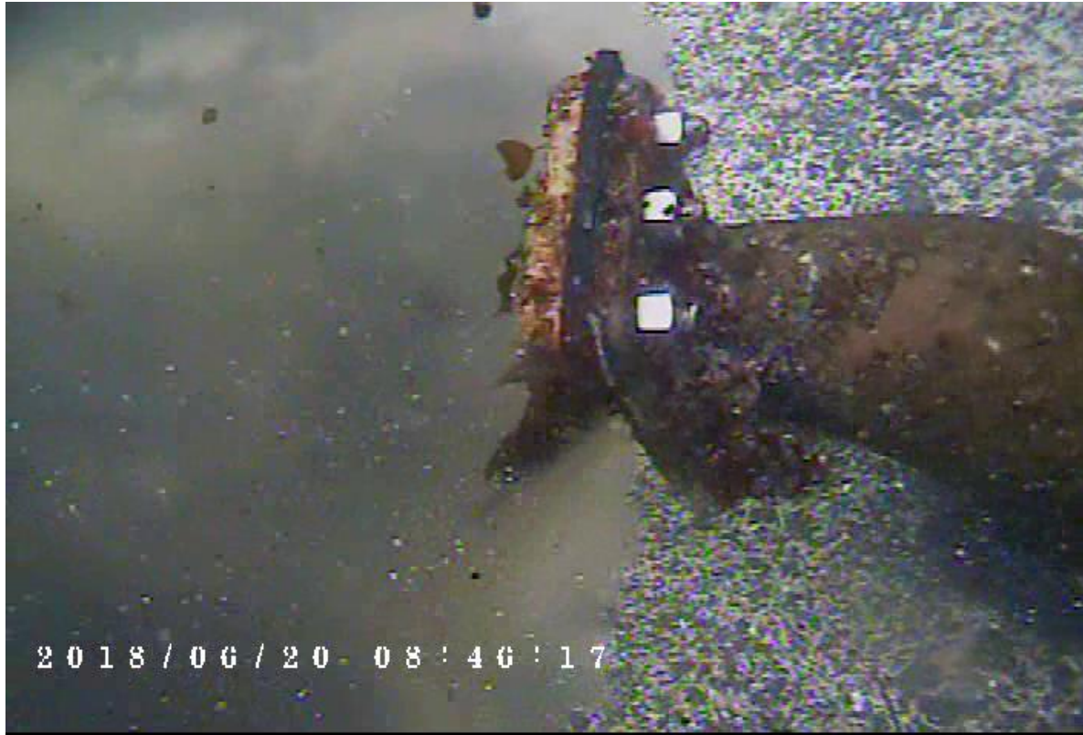
Photo 7 – Diffuser 7 showing strong flow
