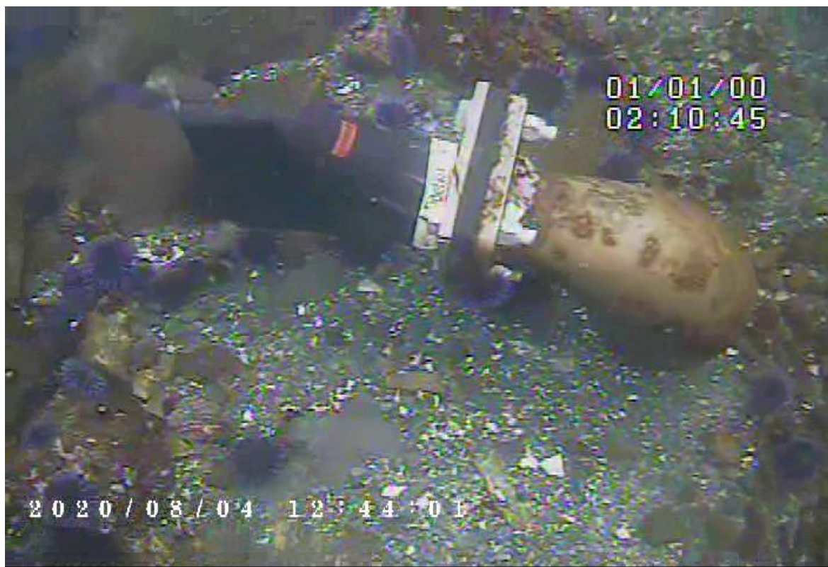
Photo 14 – Diffuser 2 showing strong flow
