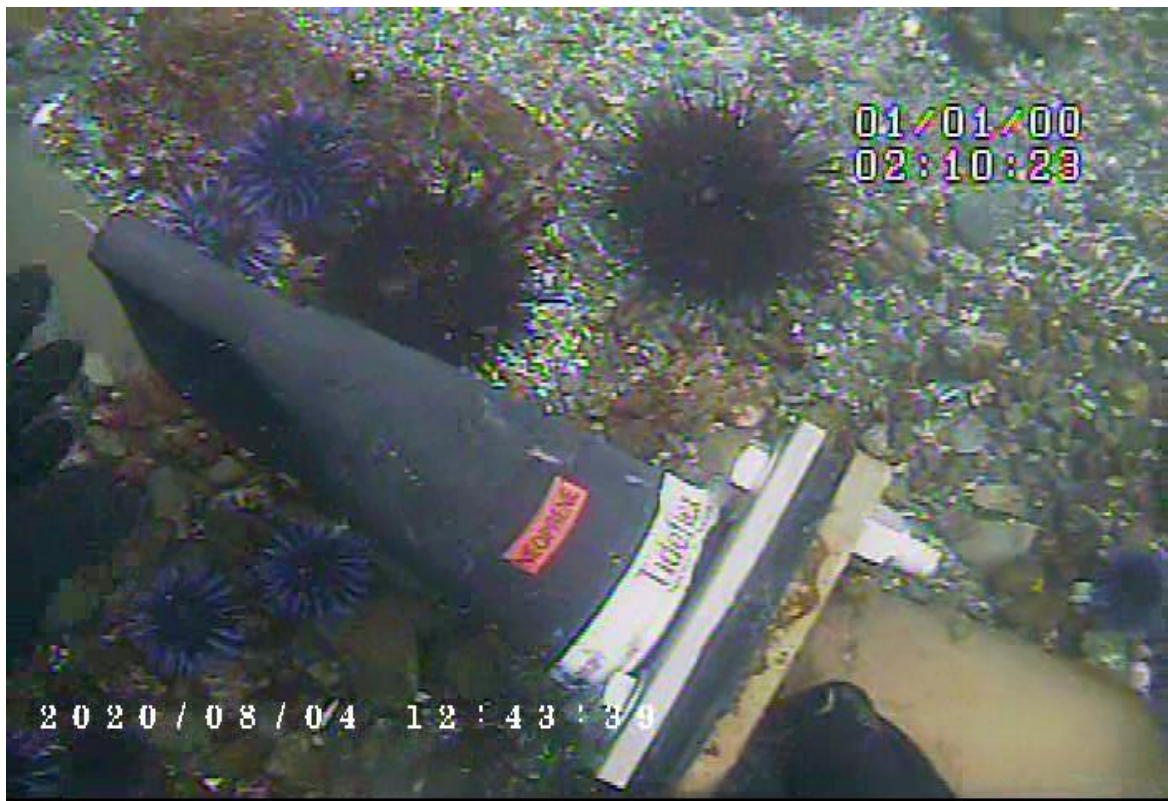
Photo 12 – Diffuser 4 showing strong flow
