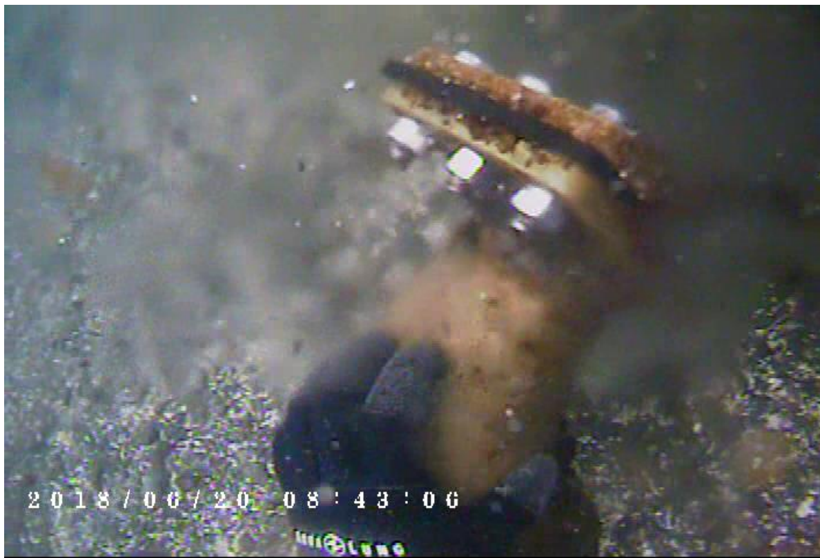
Photo 4 – Diffuser 4 showing strong flow
