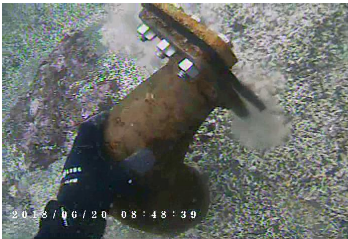
Photo 12 – Diffuser 12 showing light flow
