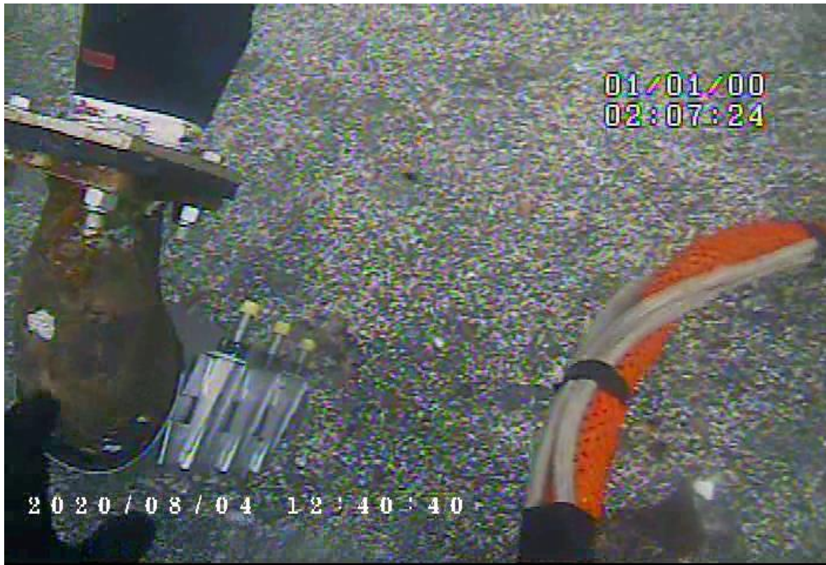
Photo 1 – Diffuser 14 clamp repair
