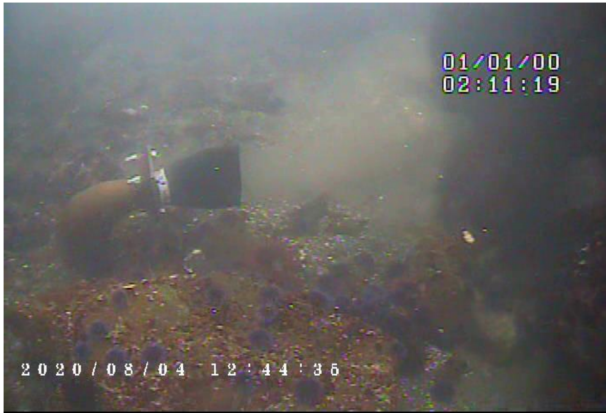
Photo 15 – Diffuser 1 showing strong flow
