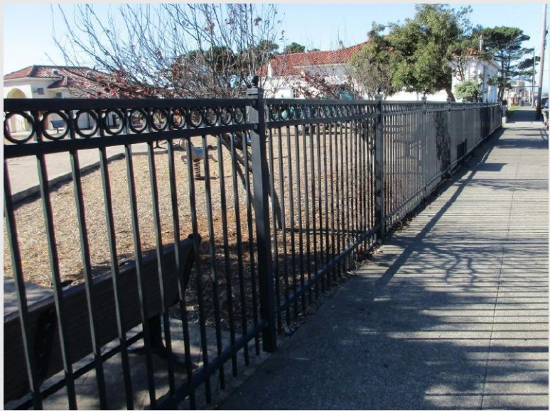
Existing fencing at Wiggly Giggly Playground.
