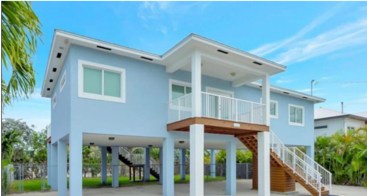
Figure 5-3: Example of Building Elevated on Piles.
