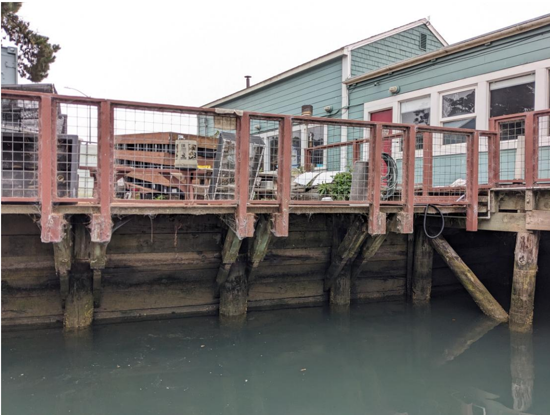
Timber wall and deck along yard looking northeast.
