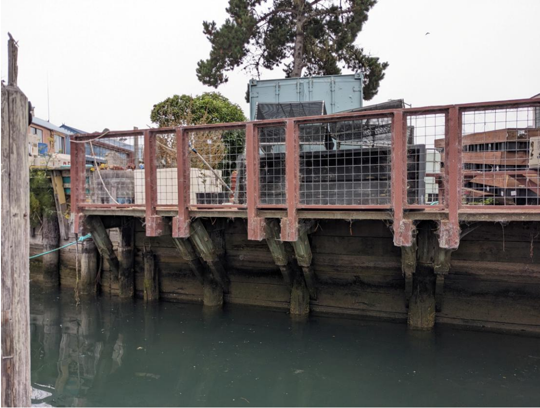
Timber wall and deck along yard looking northwest.
