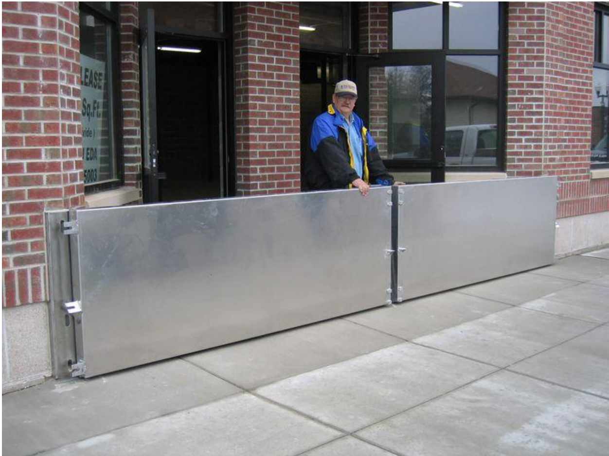
Figure 5-5: Example Barrier Utilized for Building Dry Floodproofing.
