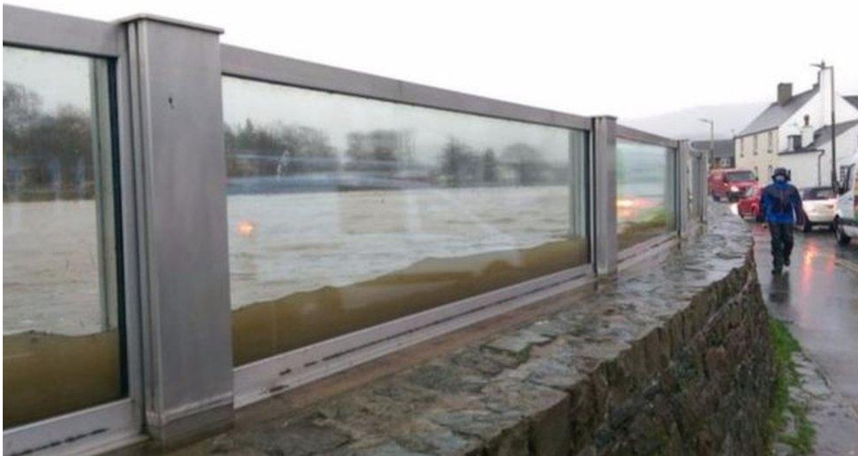
Figure 5-2: Example Flood Protection with Glass Floodwall.
