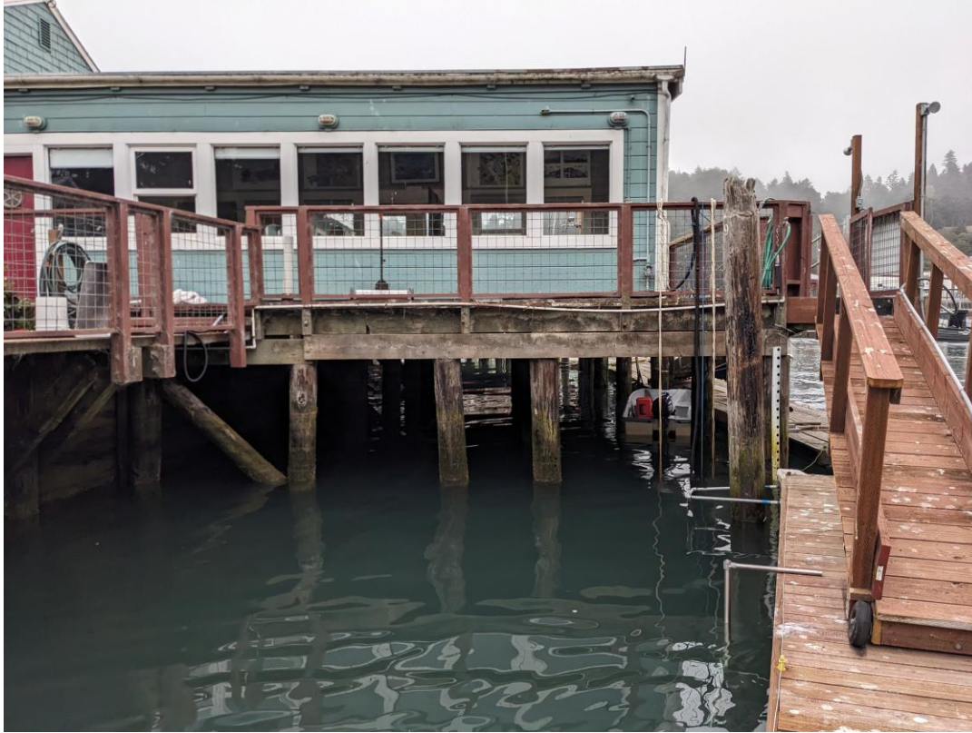
View of pile-supported and deck gangway looking east.
