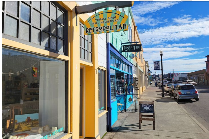
Example of the downtown streetscape
