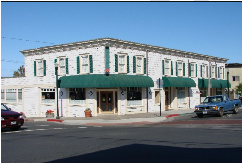
Architectural style and materials should be consistent
