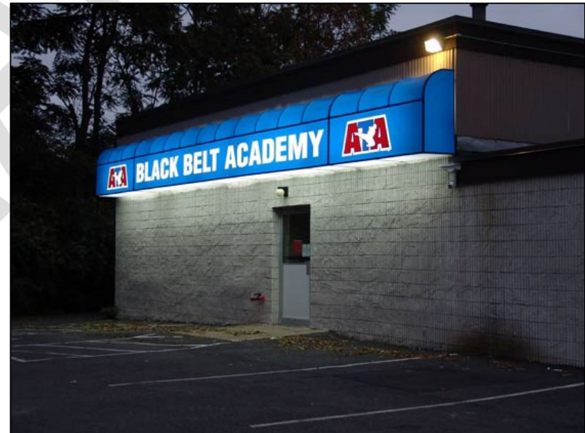
Prohibited awning sign
