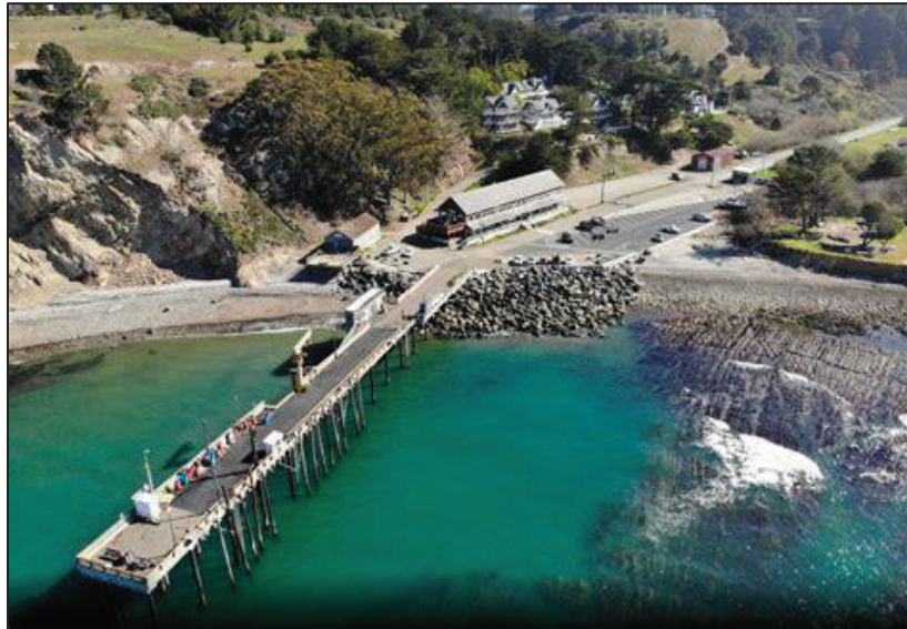
Figure 2-14 City of Point Arena Pier and Harbor
