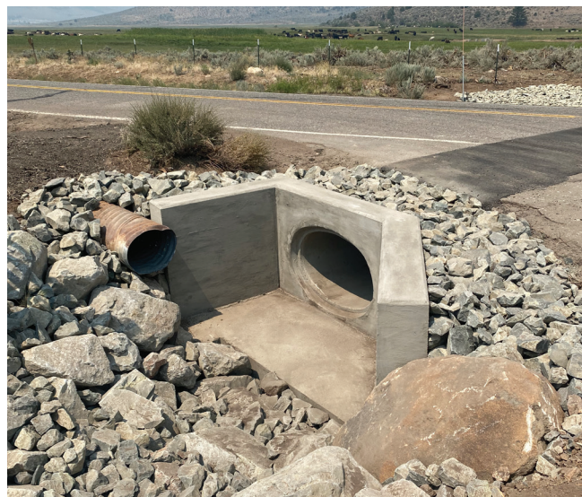
Diamond Valley & Hot Springs Rd. Erosion Control Culvert - Alpine County
