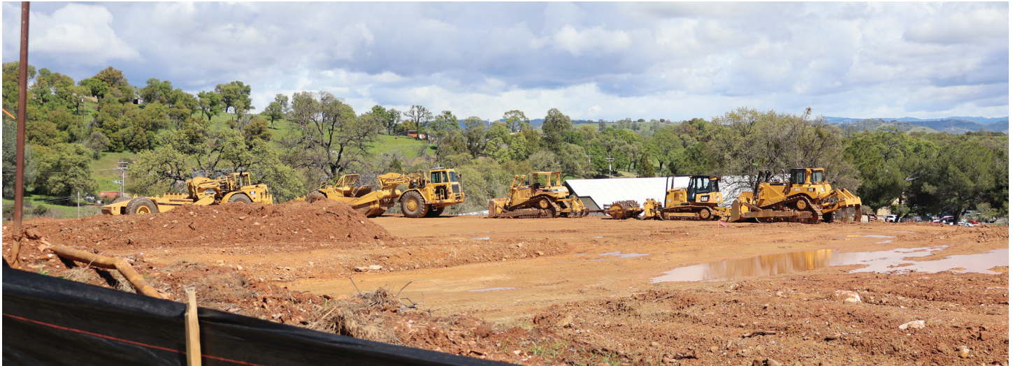
Habitat for Humanity Construction in Angels Camp
