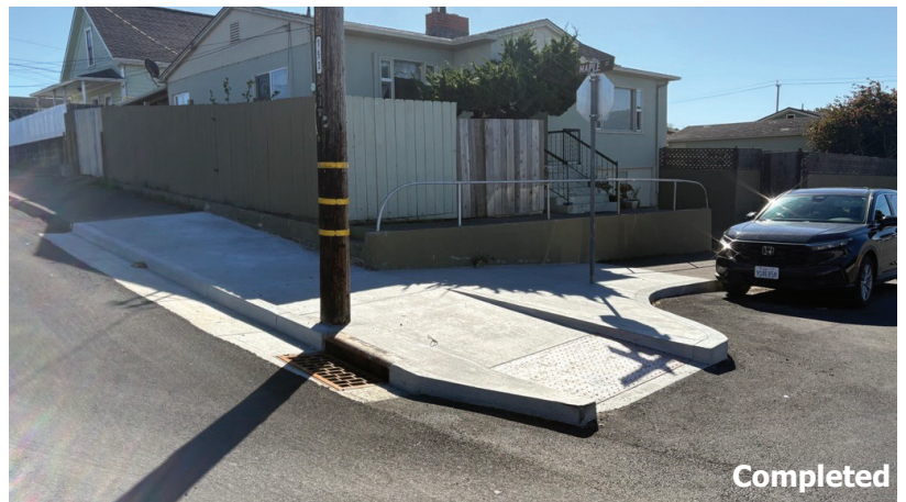
Fort Bragg - Maple at McPherson St. ADA curb ramp improvements
