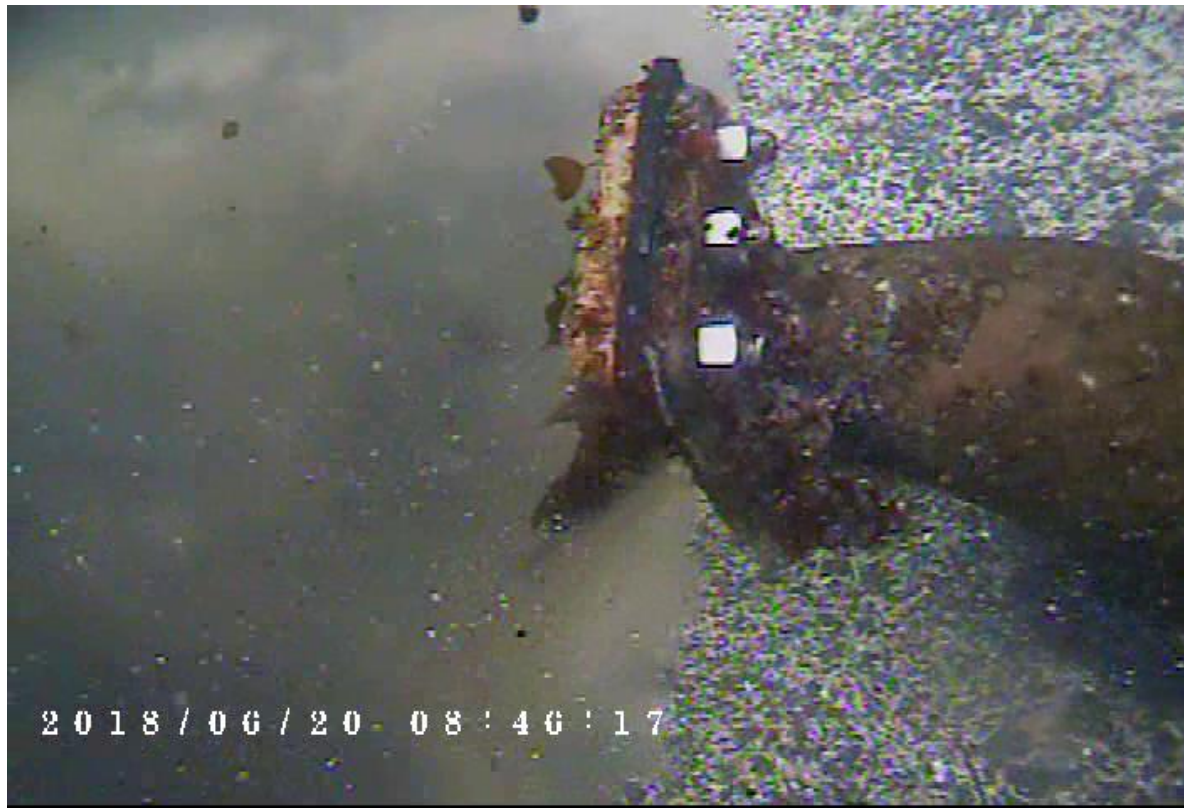
Photo 7 – Diffuser 7 showing strong flow
