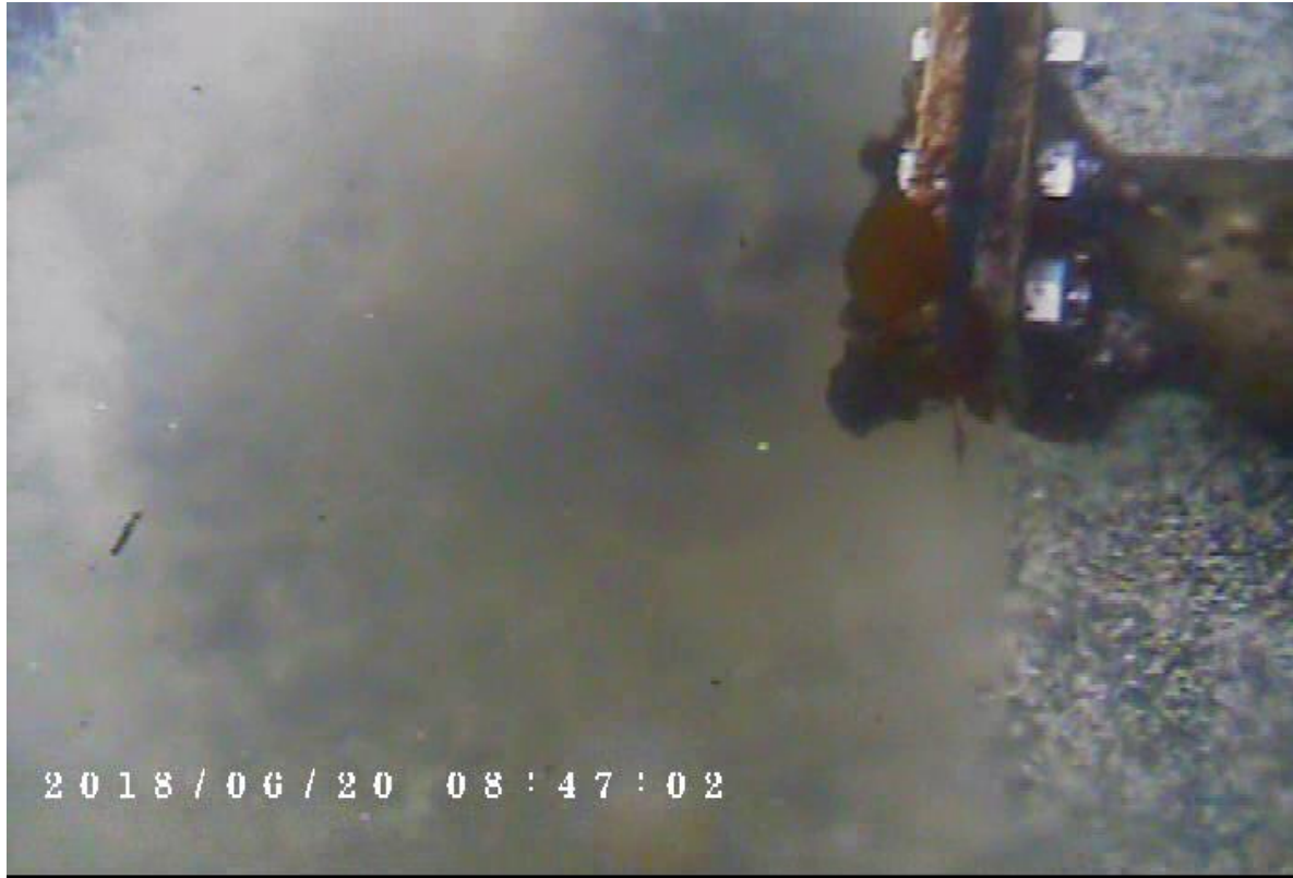
Photo 9 – Diffuser 9 showing strong flow
