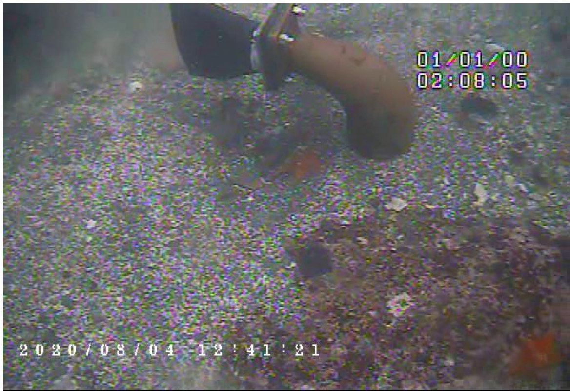
Photo 4 – Diffuser 12 showing strong flow
