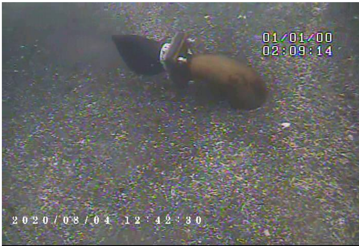
Photo 8 – Diffuser 8 showing strong flow
