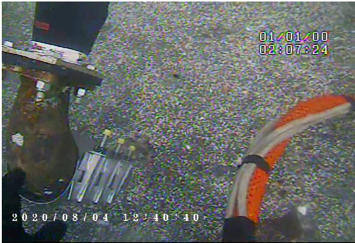
Photo 1 – Diffuser 14 clamp repair
