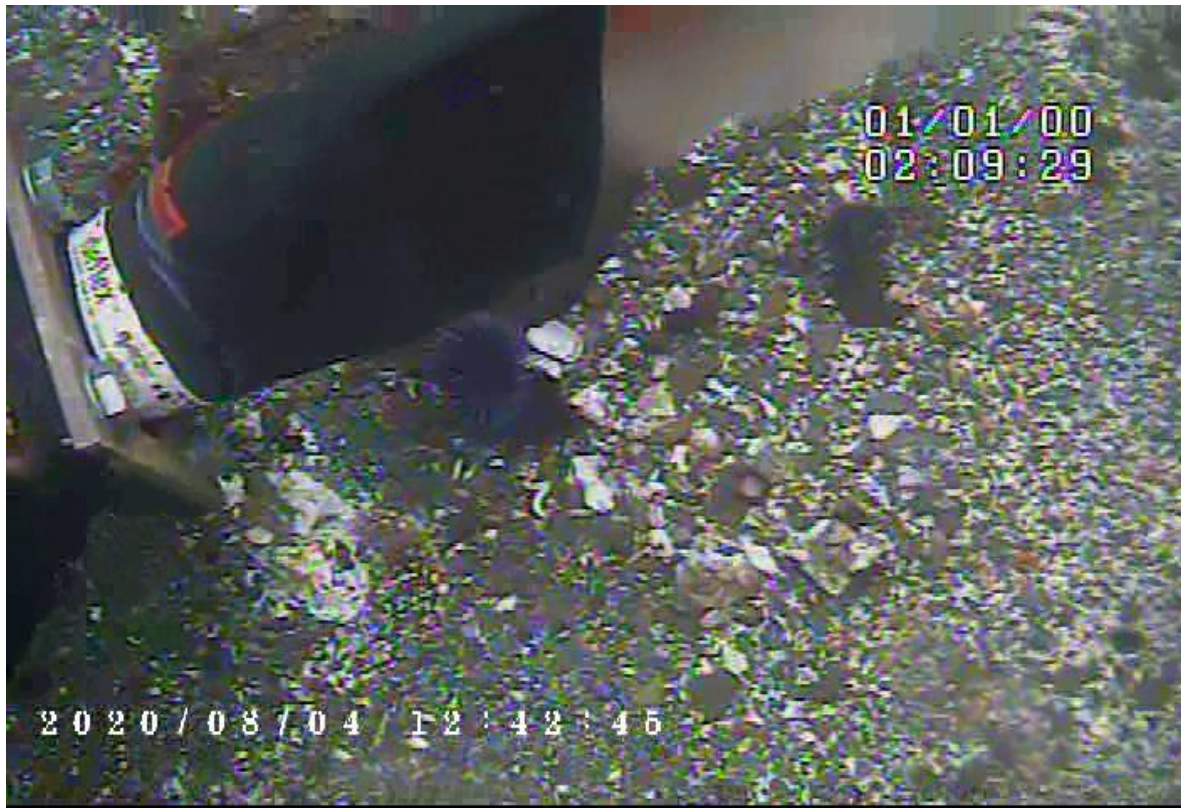
Photo 9 – Diffuser 7 showing strong flow
