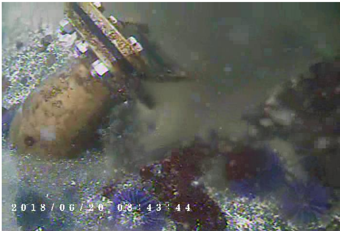
Photo 6 – Diffuser 6 showing strong flow
