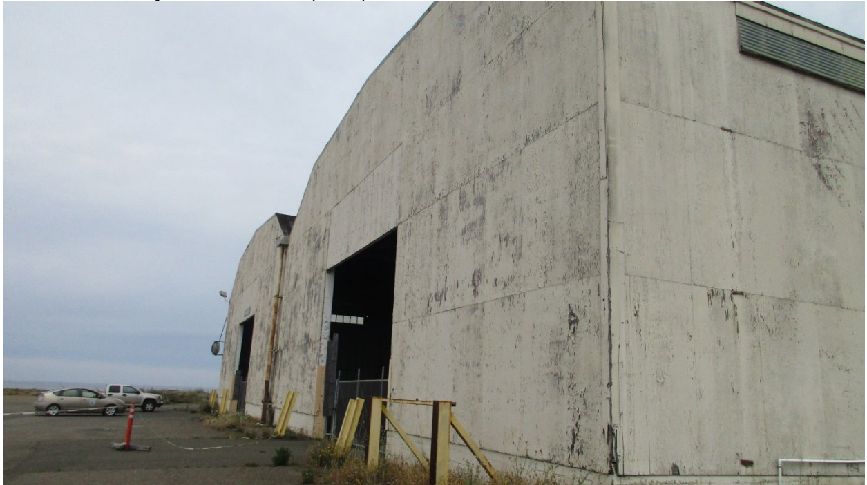
South east Corner
