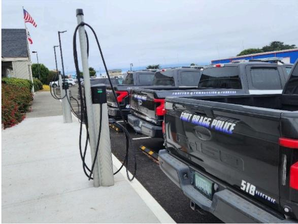
**EV Charging Stations (Police Department)** – Completed installation of four EV charging stations with six charging arms to support the City's electric patrol vehicles.
