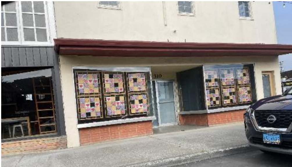
Vacant for 3+ years. 310 N Franklin Street, 1,400 SF
