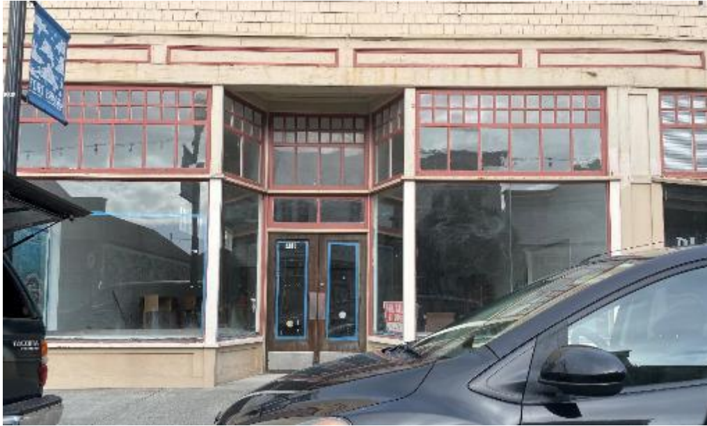
Vacant for 8+ years. 335 N Franklin Street, 2,000 SF
