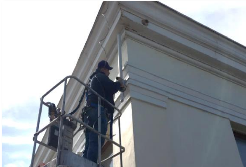
Public Wi-Fi Installation
