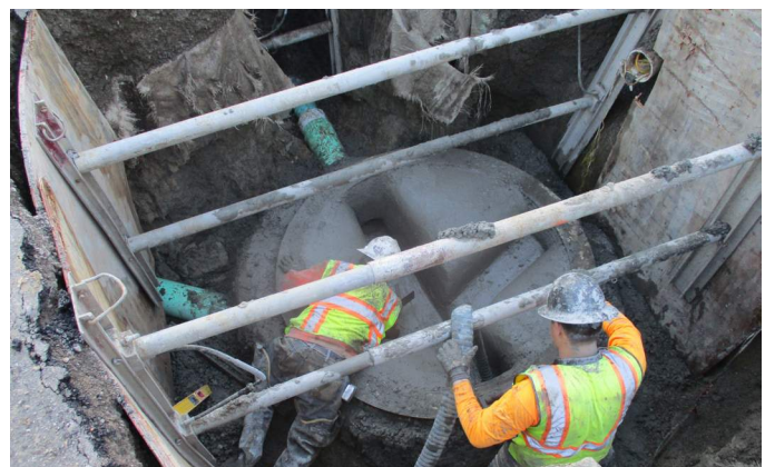
City of Cotati Sewer Collection System Repairs
