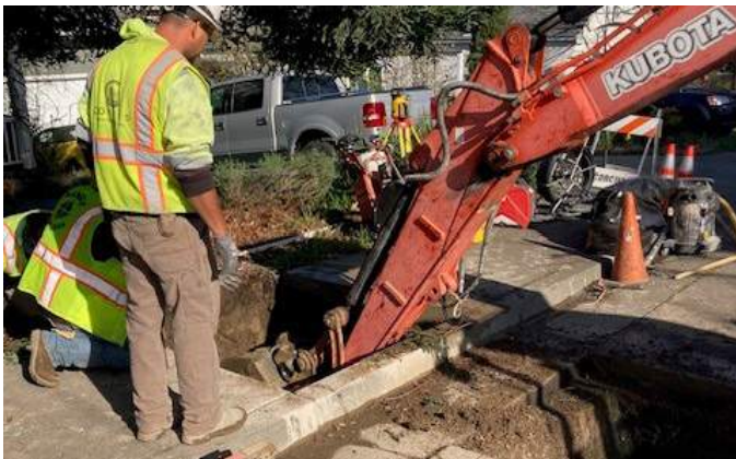
City of Cotati Cypress Avenue Sewer Repairs
