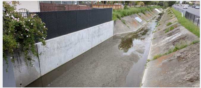
The replacement retaining wall on the Washington Creek Channel.
