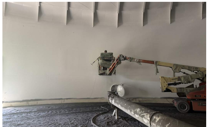
City of Petaluma Hardin Tank Rehabilitation
