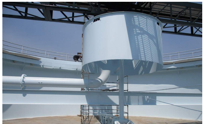
Town of Windsor AWT Clarifier No. 1 Rehabilitation
