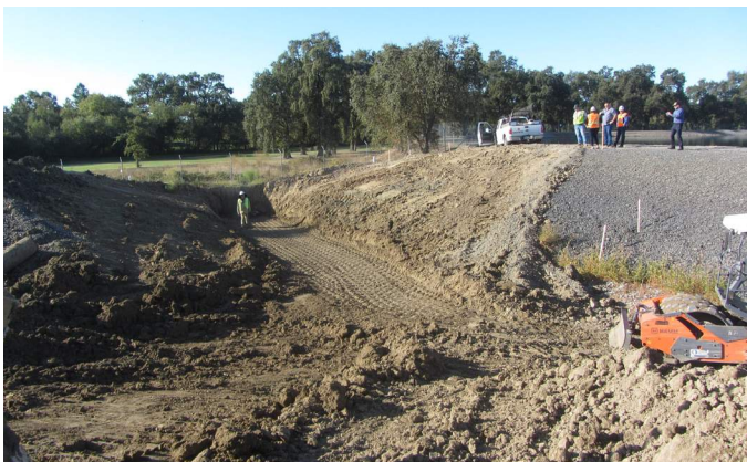
Town of Windsor Wastewater Pond 10 Leak Repair
