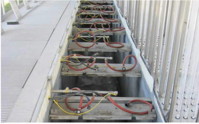
Town of Windsor Wastewater Treatment UV Replacement
