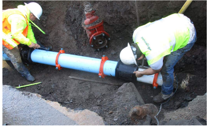
City of Santa Rosa Slater and Lewrosa Sewer & Water Replacement
