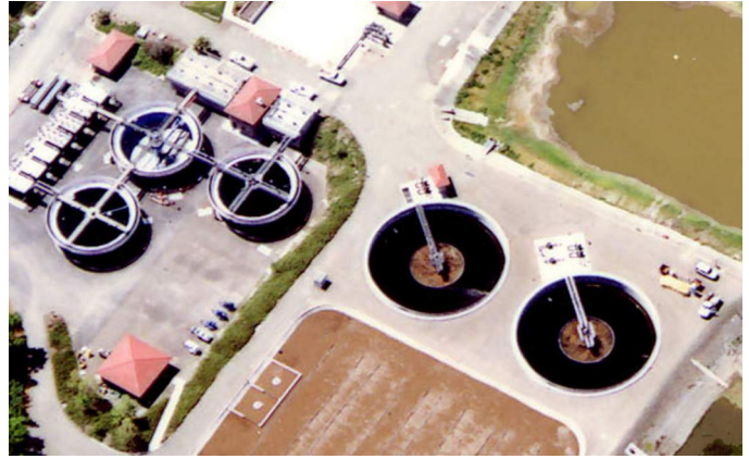
Aerial View of the Town of Windsor Wastewater Treatment Plant
