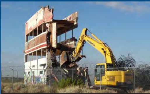
Abatement and demolition at the Beeline Dragway, Scottsdale, AZ.
