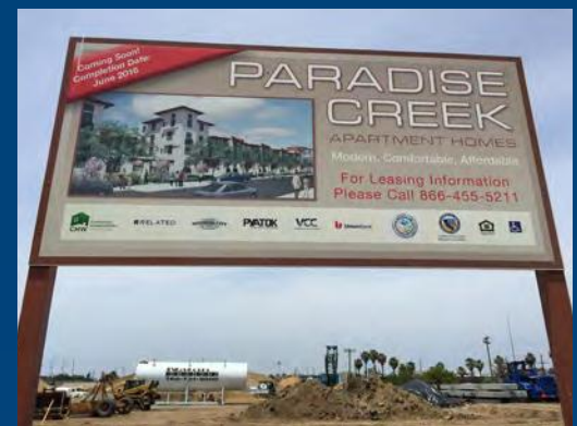
Paradise Creek Apartment Homes are the first sustainably redesigned affordable homes in West-side neighborhood in the City of National City.
