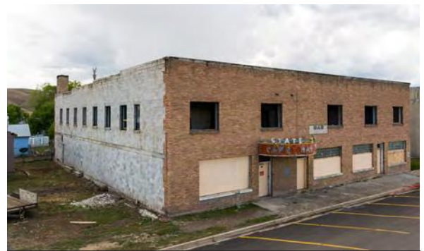
The State Hotel in Carlin, NV was assessed under an EPA grant, and asbestos abatement and building demolition will be funded through Nevada's 128(a) grant. The city plans to reuse the site as a community garden.
