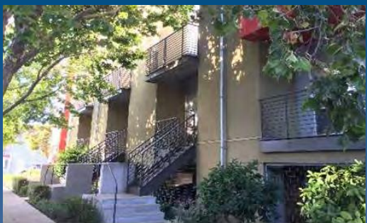
Developers of Emeryville's GreenCity Lofts used a low-interest revolving loan to clean up the site for this mixed-income multifamily development.
