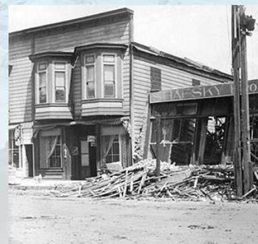
Damage from the Great Earthquake
