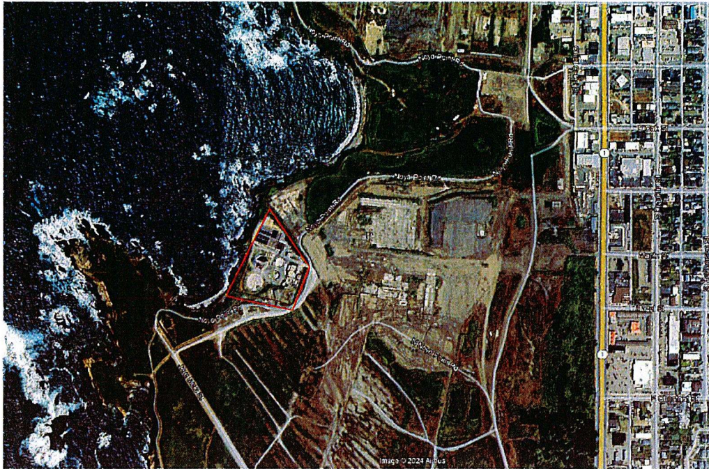
Figure 1: Wastewater Treatment Plant Aerial Image 2
