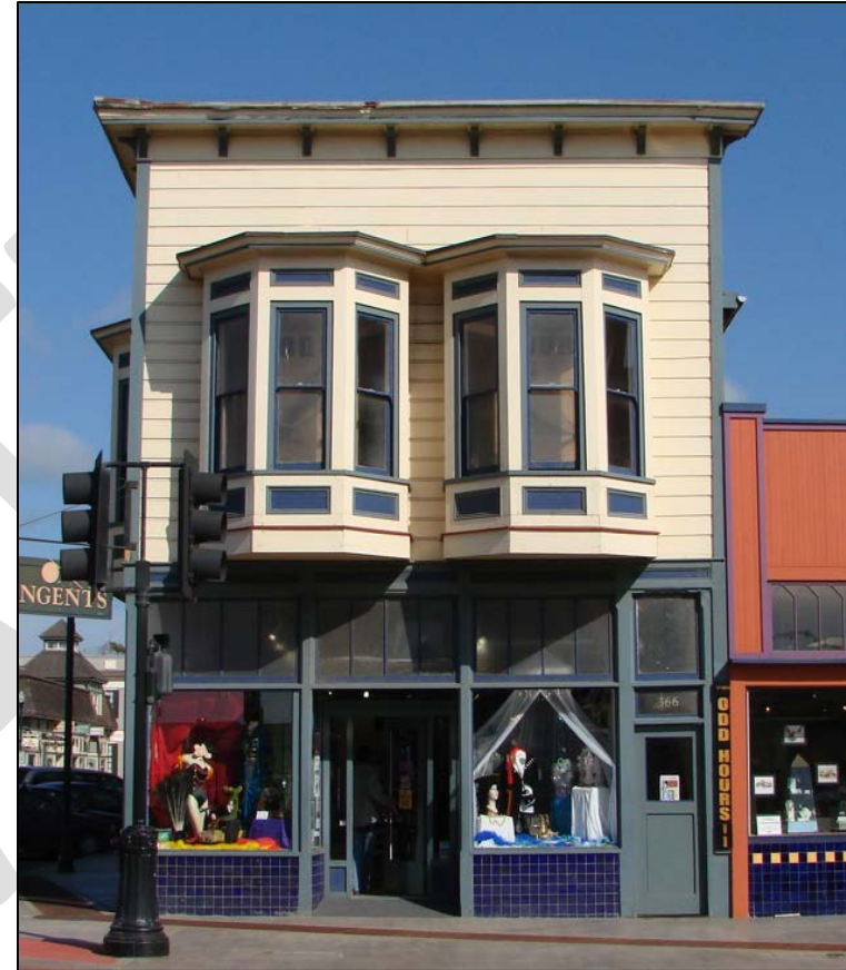
Example of the downtown streetscape
