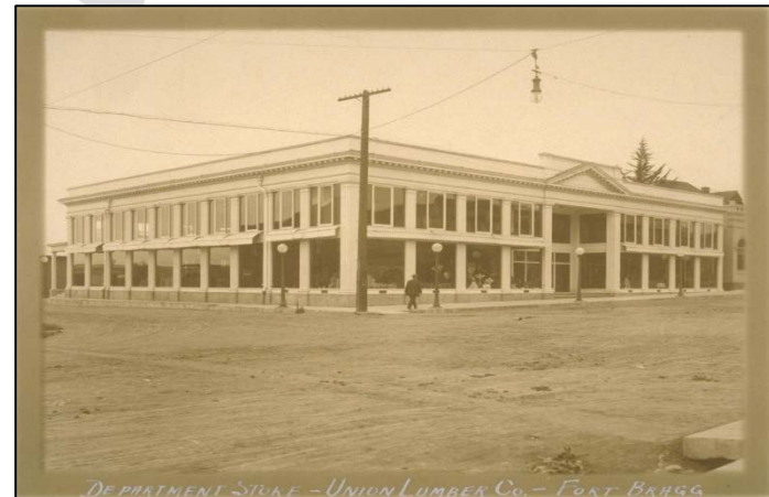
Use of recesses are strongly encouraged to provide protection for pedestrians. (Union Lumber Company Store Early 1900s)
