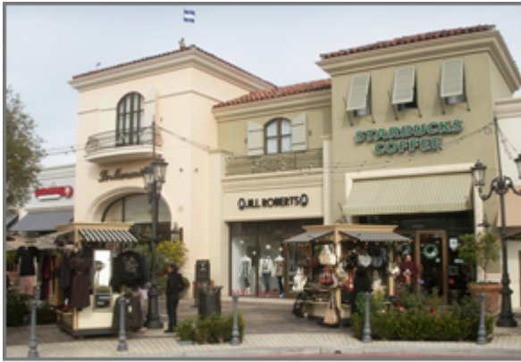
Varied roof forms, projecting balconies, and awnings help divide building mass into smaller components
