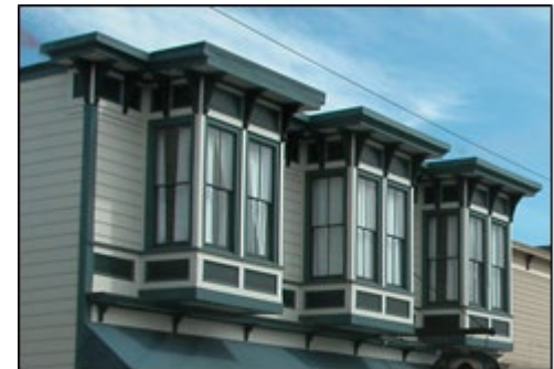
Wood siding is the predominant downtown building material
