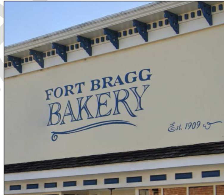
Example of an acceptable ghost sign
