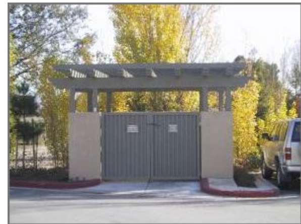
Trellis provides continuity with surrounding architectural elements
