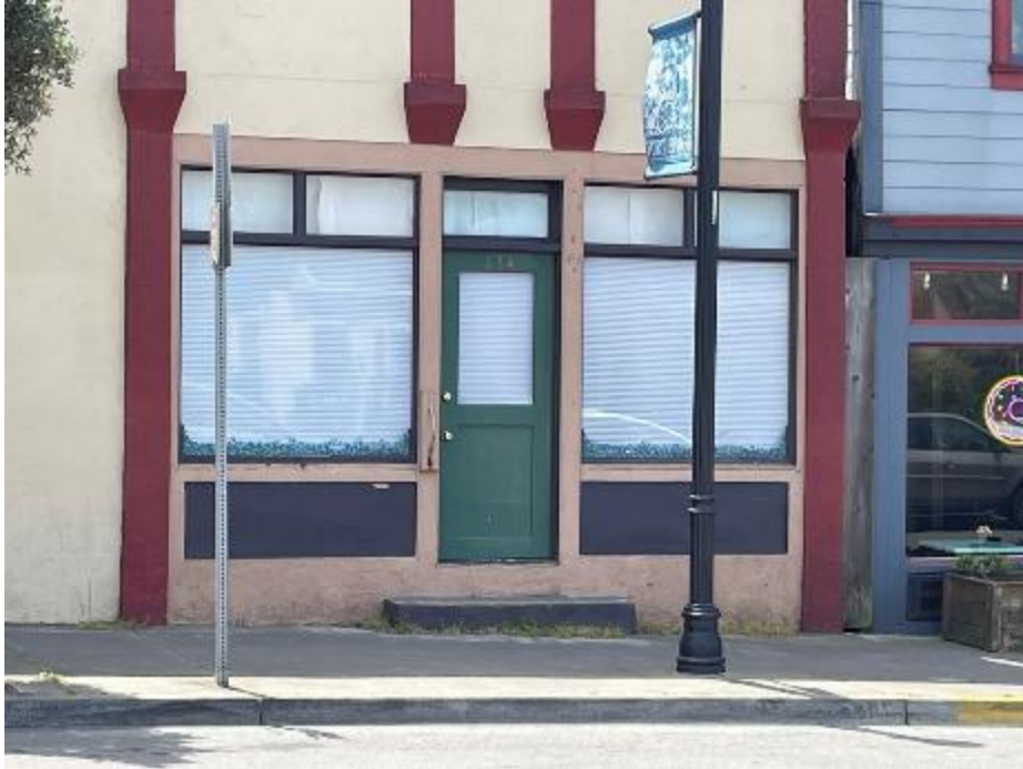
Former consignment store, vacant 134 E Redwood Ave., 600 SF
