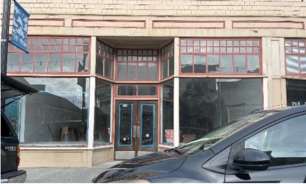
Vacant for 8+ years. 335 N Franklin Street, 2,000 SF
