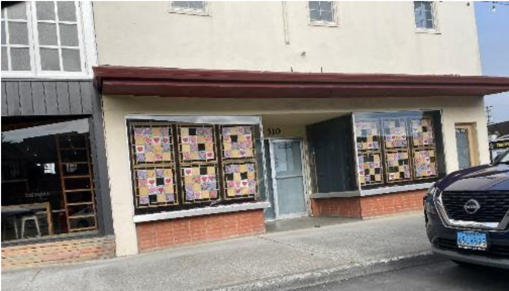
Vacant for 3+ years. 310 N Franklin Street, 1,400 SF
