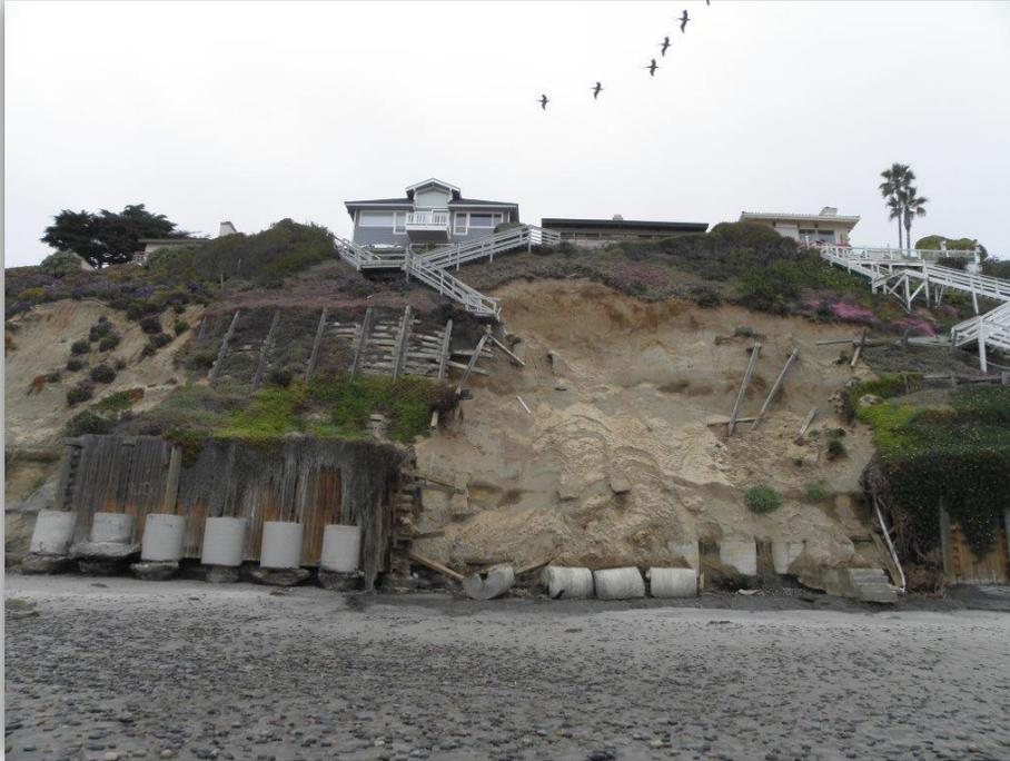
Figure 19. Photo depicting eroding bluff and exposed caissons in Encinitas, CA. (Photograph by Lesley Ewing)
