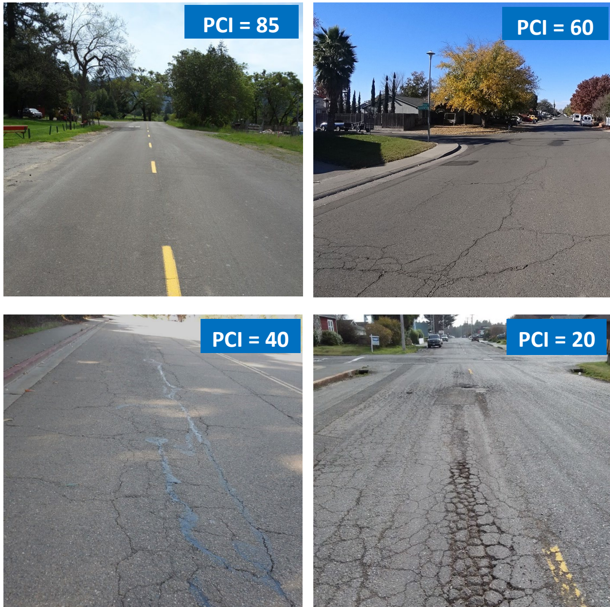
Figure 2. Examples of Streets with Different PCIs
