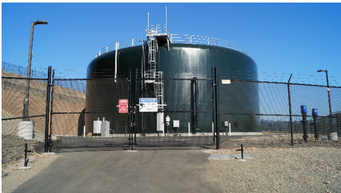
Tank 8, Rohnert Park
