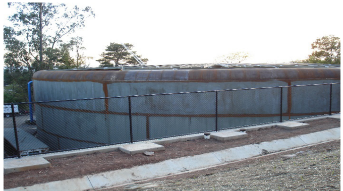
Proctor Heights tanks, Santa Rosa
