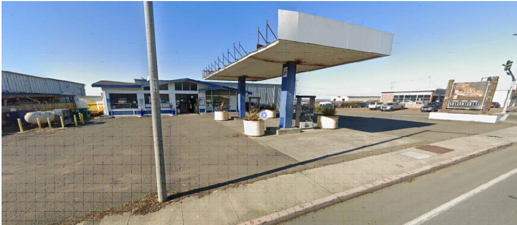
Figure 1: Photo illustrating damaged canopy.
