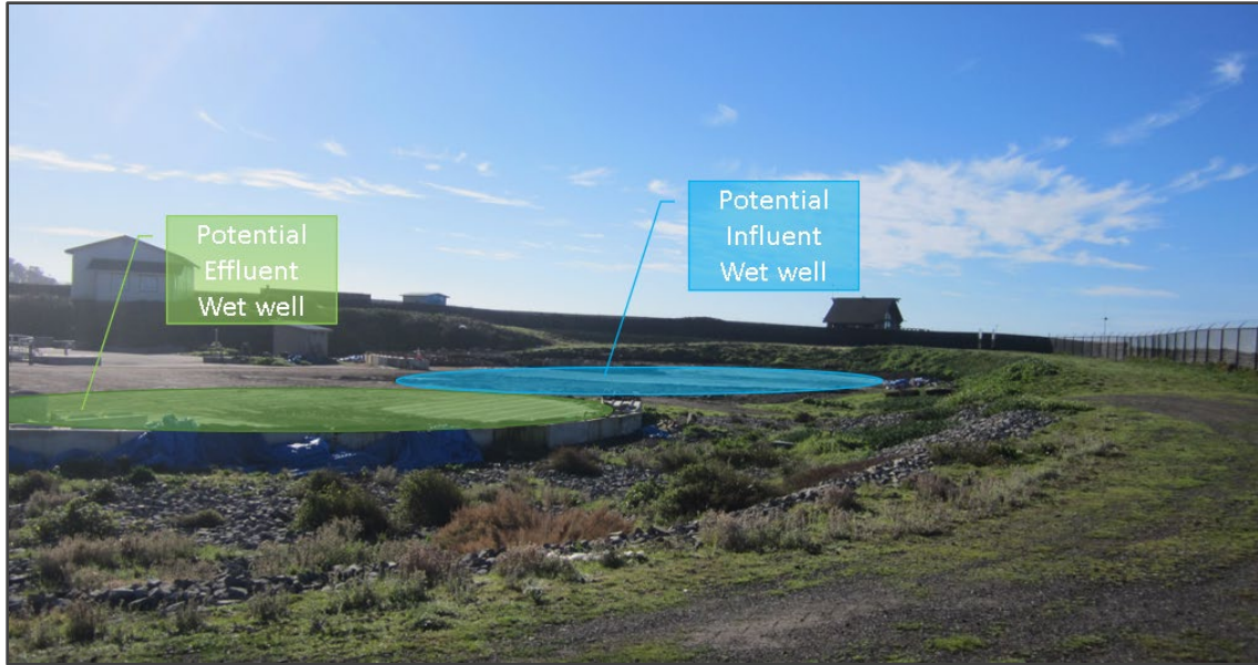
Figure 6-1. Former Trickling Filters at the City of Fort Bragg Wastewater Treatment Facility.
