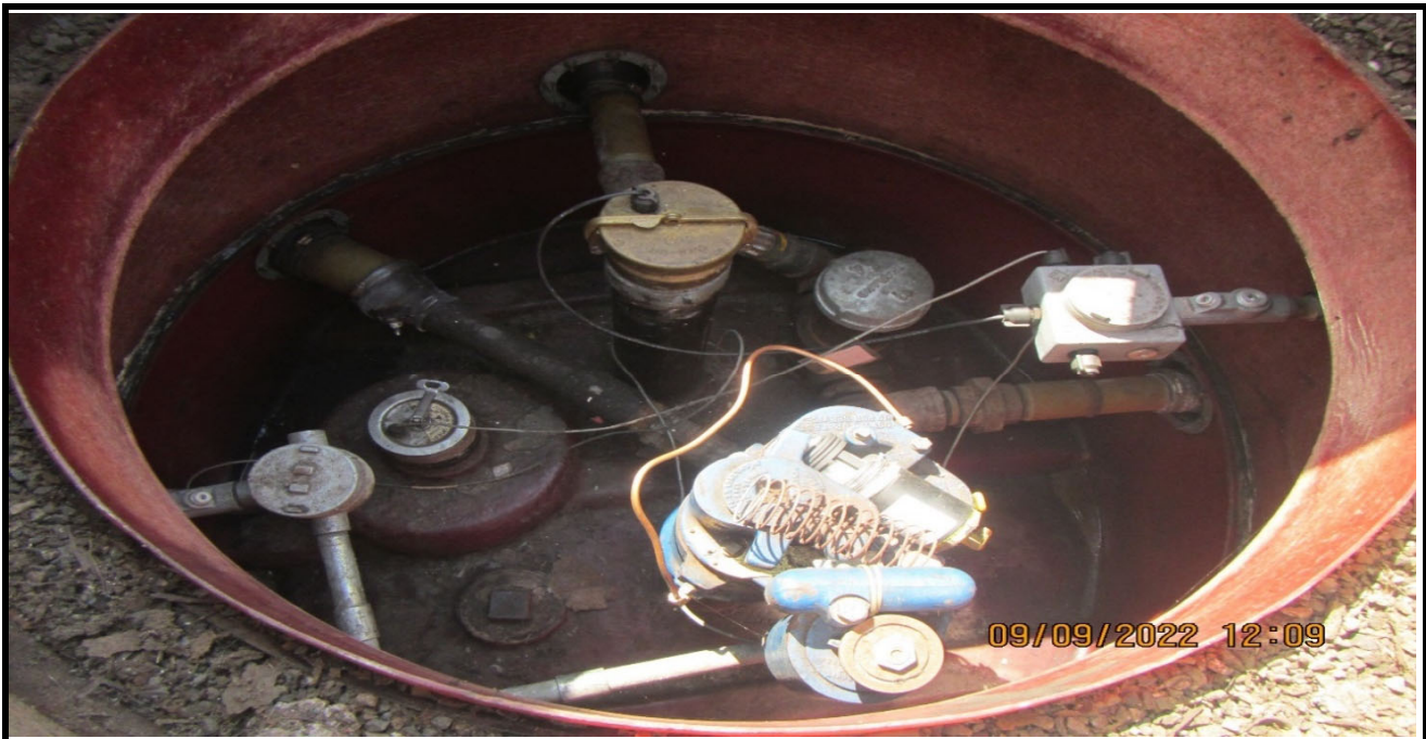
Photo No. IMG_0017-Turbine Sump of tank two, eastern tank
