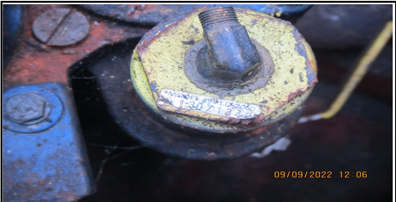
Photo No. IMG_0010-LLD inside tank one, western tank turbine sump
