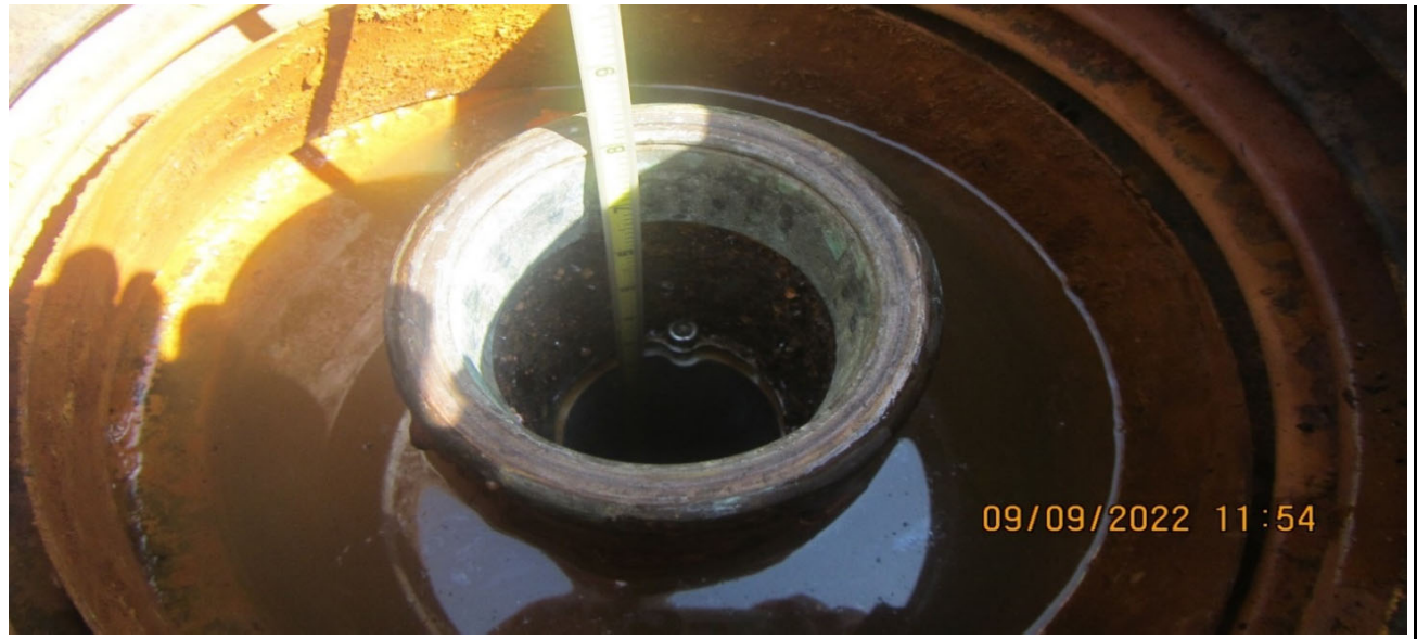
Photo No. IMG_0008-Tape measurement of product level inside tank one, western tank.
