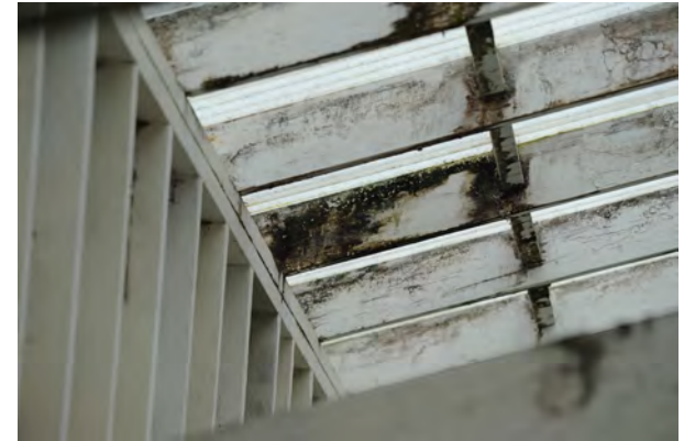
ATRIUM FRAMING, POOL
