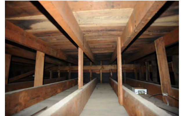
FRAMING ABOVE NORTH WING OF CITY HALL EAST
