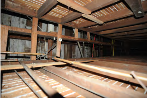
LOW FRAMING AT SOUTH WING OFF POOL
