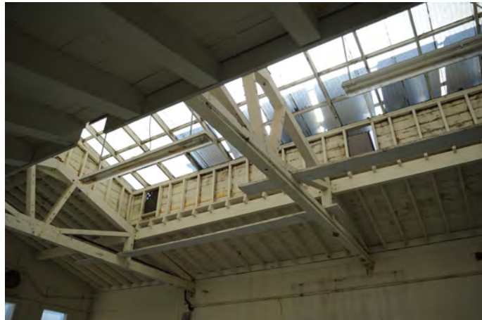
ATRIUM AND WOOD TRUSSES IN POOL BUILDING
