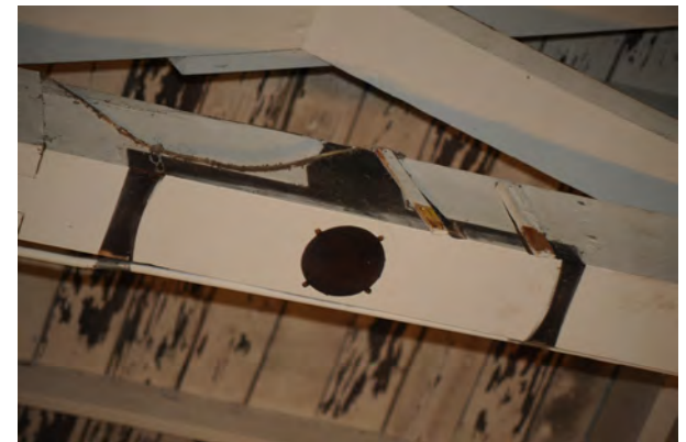
ROOF TRUSS AT GYMNASIUM
