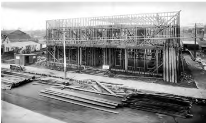
VIEW FROM FRANKLIN - BUILDING UNDER CONSTRUCTION
