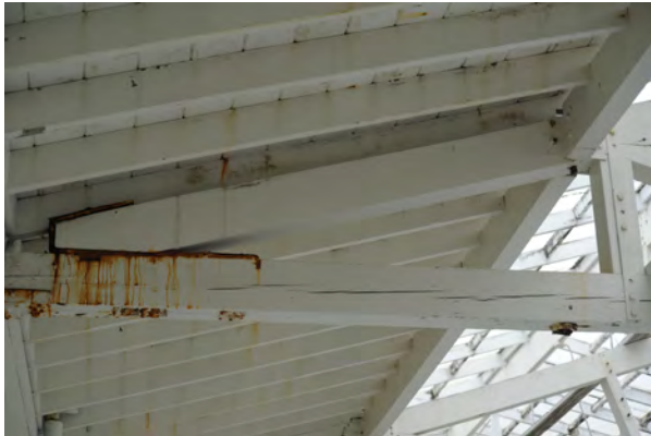
POOL TRUSS AND LOW BAY FRAMING
