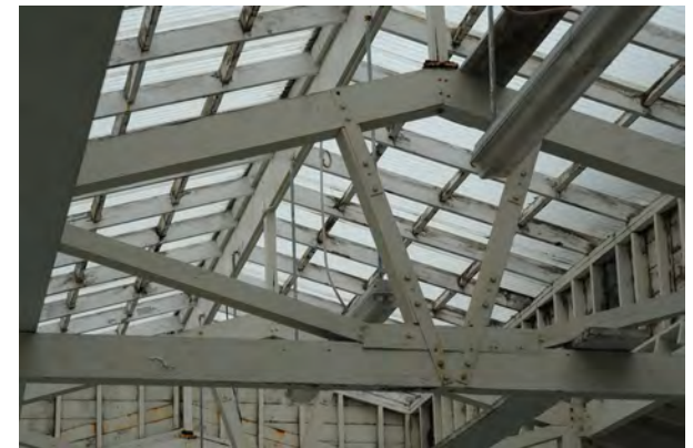
TRUSS AND ATRIUM AT POOL
