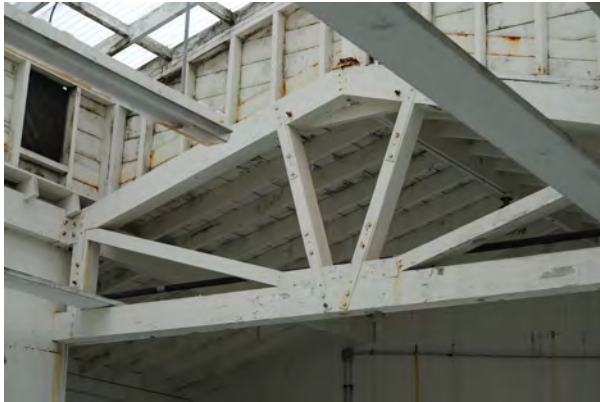
TRUSS AND ATRIUM IN POOL BUILDING
