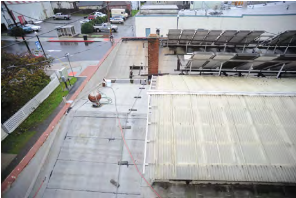
VIEW FROM ROOF LOOKING SOUTH
