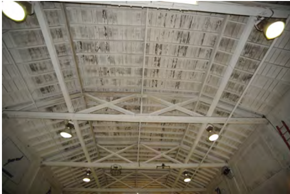
TRUSS AND GYMNASIUM
