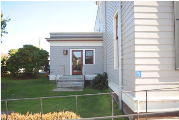
VIEW FROM FRANKLIN STREET TO NORTH ELEVATION
