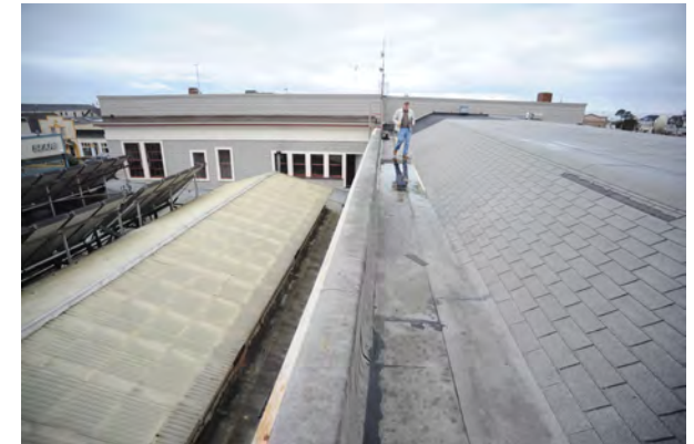
HIGH ROOF ABOVE GYMNASIUM WITH POOL ATRIUM BELOW
