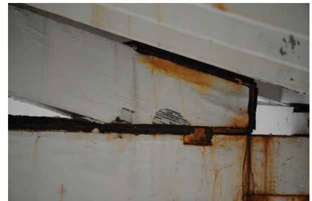
TRUSS AT WALL, POOL
