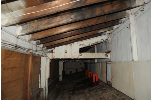
FRAMING AT SOUTH WING, LOW BAY SPACE
