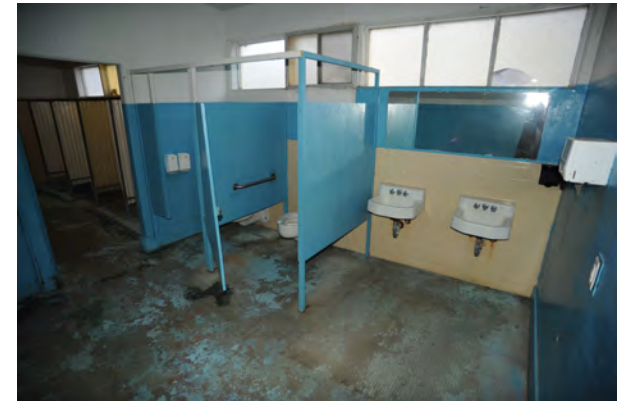
SHOWER/RESTROOM FACILITIES OFF GYMNASIUM
