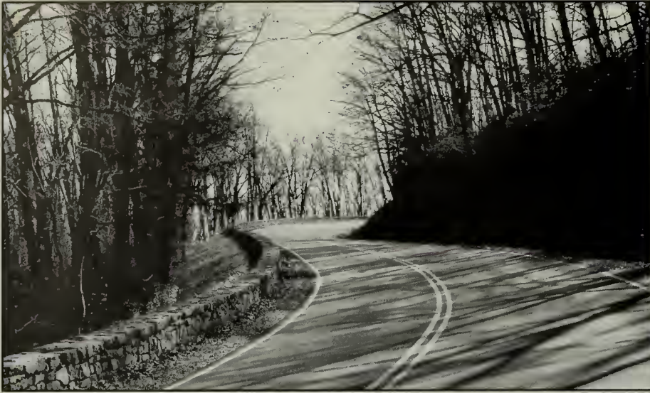
A 75-mile portion of Skyline Drive at Shenandoah National Park overlooking the Blue Ridge Mountains of Virginia required the rehabilitation of a 22"-high, dry-laid stone wall [opposite]. The new wall was built to a height of 27" whereas code normally requires a height of 36". The wall was constructed of precast concrete, clad with split stone and mortar joints [center]. To achieve visual compatibility, recessed mortar joints were arranged in a random pattern [bottom]. (courtesy NPS and Paul Daniel Mariott)
