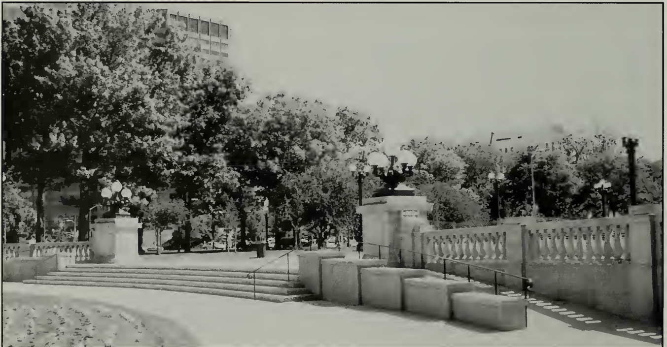
This accessibility solution for Denver, Colorado's Civic Center, retains character-defining features and visual relationships. The new ramp is not visible from the plaza's east-west vista and, thus, respects its symmetrical design. (author, 1993)
