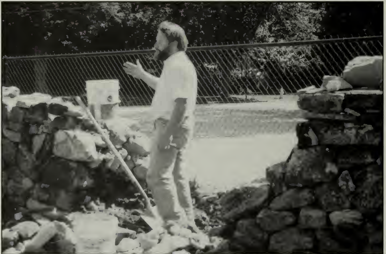
A section of a historic wall at Stan Hywet Hall in Akron, Ohio, was in need of restoration. Here, the limited replacement of a section of the wall was undertaken utilizing surviving stone and stones that matched the old in form, size, and color. Compatible substitute material could also have been used (author, 1993)
