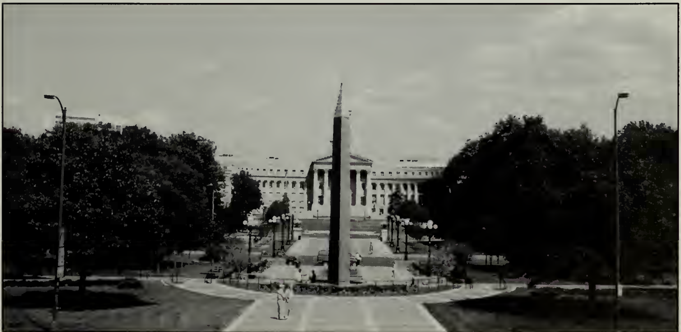
The addition of this war memorial to the Civic Center in downtown Denver, Colorado, compromised the character-defining visual and spatial relationships of S. R. DeBoer's 1924 design for the plaza. (author, 1993)
