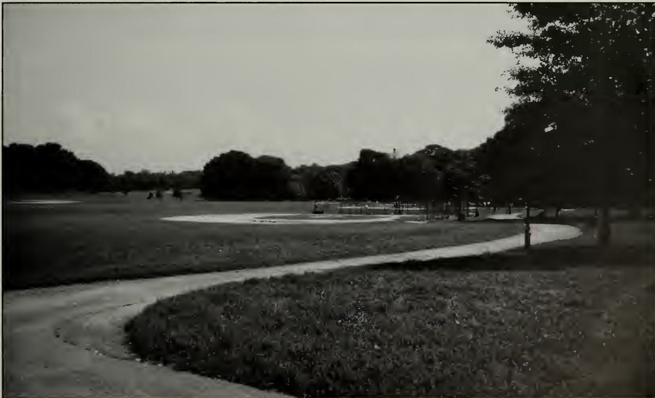
As part of a comprehensive rehabilitation project for Prospect Park's Long Meadow, in Brooklyn, New York, a non-historic ball field was relocated to minimize its impact on the great greensward. Here, the backstop and associated fences are realigned along a woodland edge. The new fencing is limited in scope, and painted black to recede into the viewshed. (Prospect Park Alliance)
