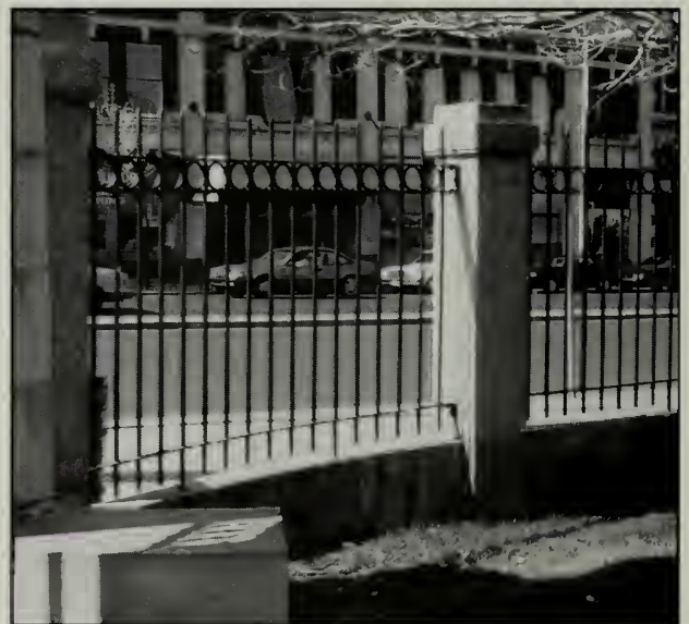
A section of the wall surrounding the Dorchester North Burying Ground in Massachusetts was in a state of advanced deterioration. [top] Rather than reconstruct the failing wall along the main entrance area, only its piers were replaced. [bottom left] The area of wall between these piers was replaced with an iron fence. [bottom right] This approach was selected to improve the perceived safety and security of the burial ground, thus allowing for visual access into the burial ground, where it was previously enclosed. (author, 1993 and Boston Parks)
