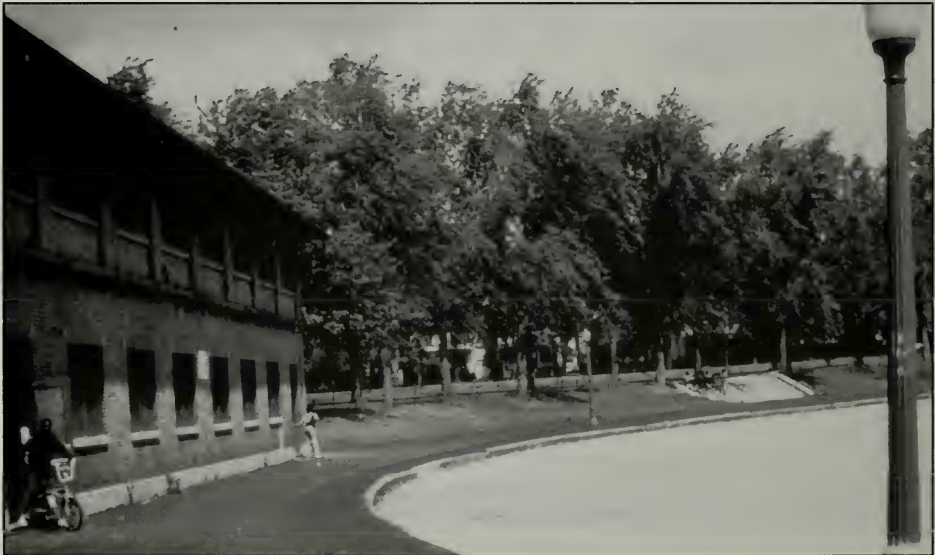
Prior to rehabilitation project work, this five-acre wading pool in Martin Luther King Park in Buffalo, New York, was evaluated to understand its historic design and use. It was determined that, although the pool and poolhouse were in disrepair, they possessed a high level of integrity. (LANDSCAPES)
