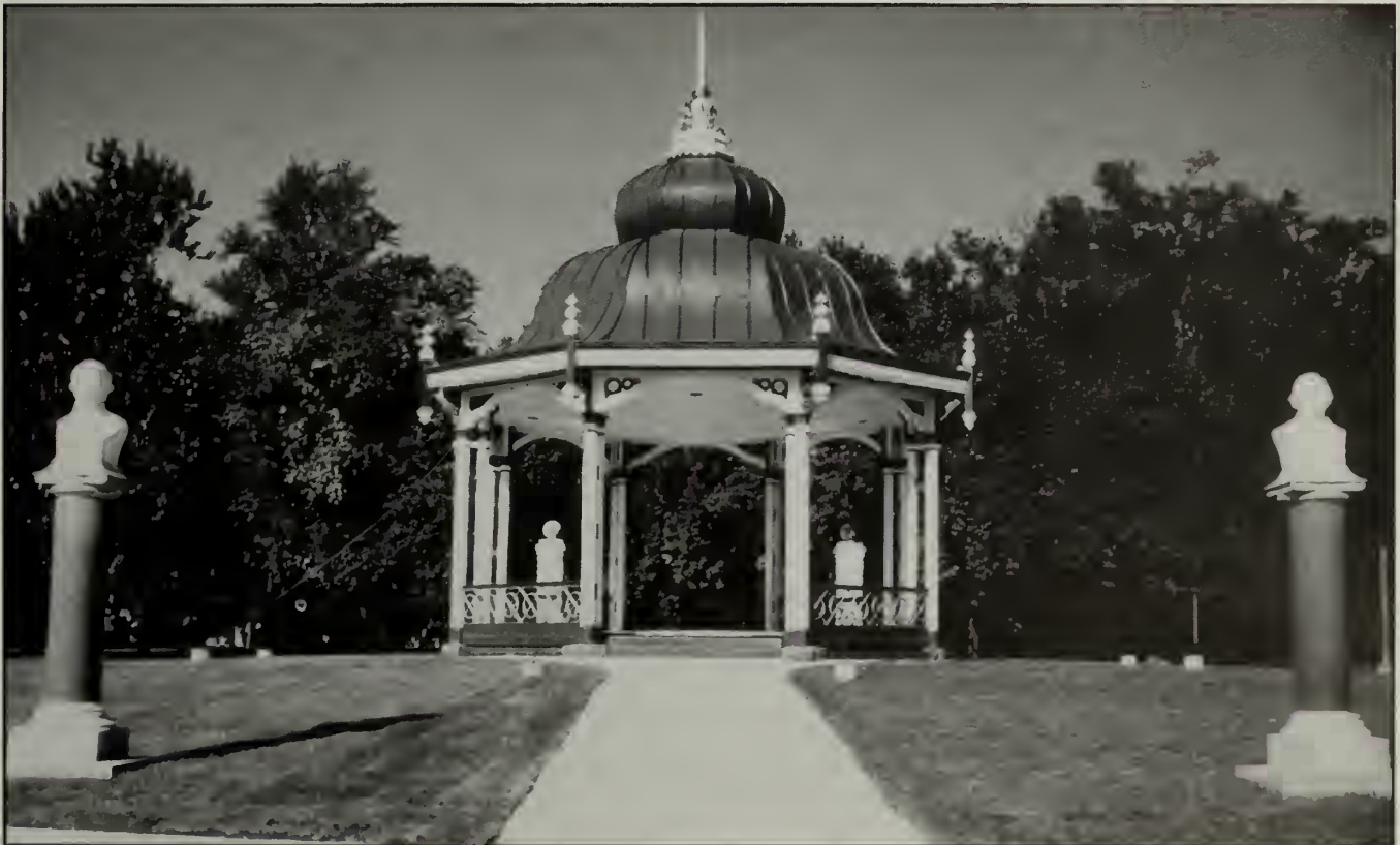
The area known as the music pavilion at Tower Grove Park in St. Louis, Missouri, had been badly deteriorated including its central pavilion, marble busts, radiating walks, lawn areas and curbing. Utilizing photographic documentation, [top] the pavilion [opposite top right] and its associated landscape were restored to portray the pavilion as it would have appeared at a certain time. For example, the marble busts of eminent composers were replaced with pre-cast concrete replicas of the originals [bottom, foreground]. (Tower Grove Park)
