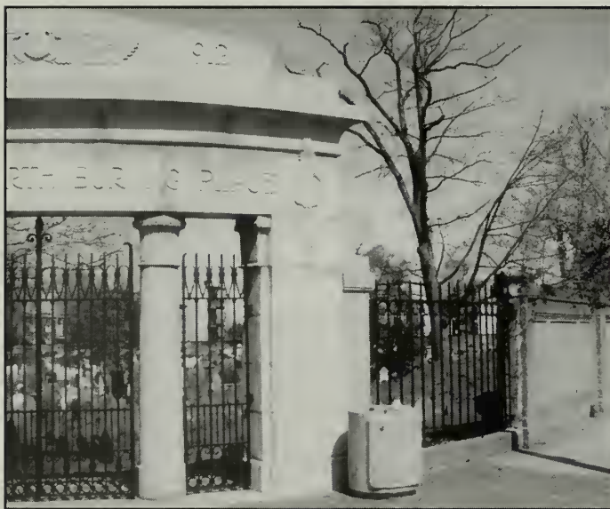
A section of the wall surrounding the Dorchester North Burying Ground in Massachusetts was in a state of advanced deterioration. [top] Rather than reconstruct the failing wall along the main entrance area, only its piers were replaced. [bottom left] The area of wall between these piers was replaced with an iron fence. [bottom right] This approach was selected to improve the perceived safety and security of the burial ground, thus allowing for visual access into the burial ground, where it was previously enclosed. (author, 1993 and Boston Parks)
