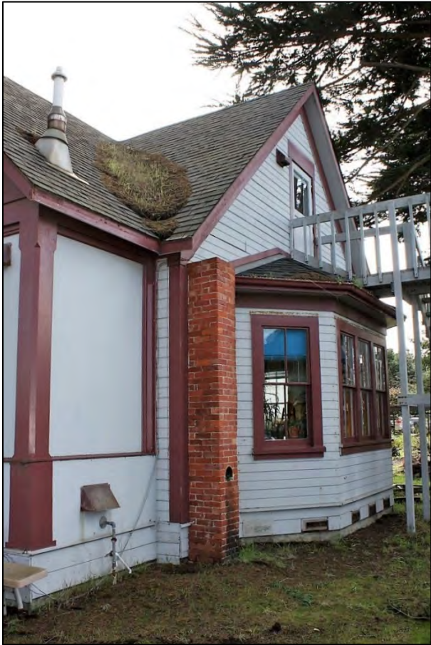
West side façade, looking south
