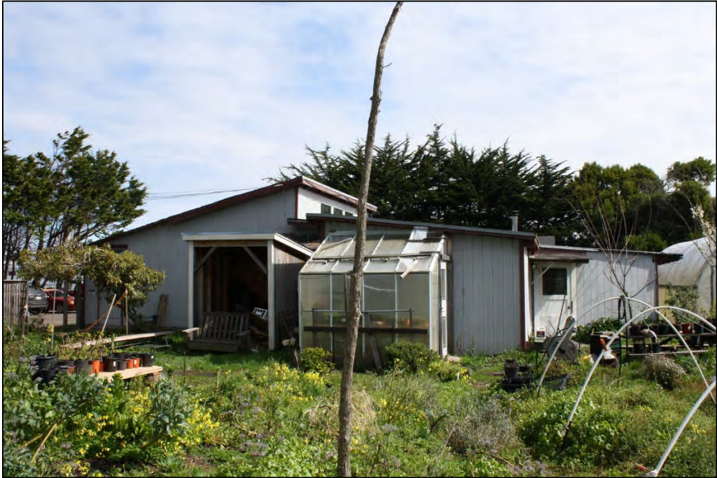
Rear (west) façade, south end, looking east
