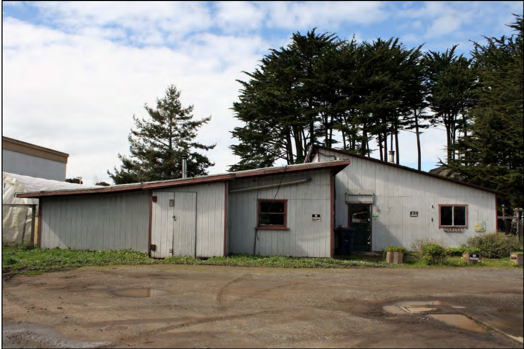
Front (east) façade, looking west
