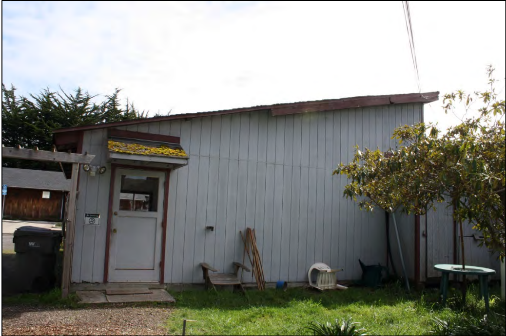
Rear (south) façade, north end, looking east
