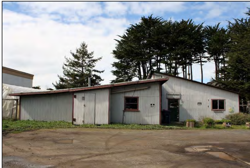
East façade, looking west
