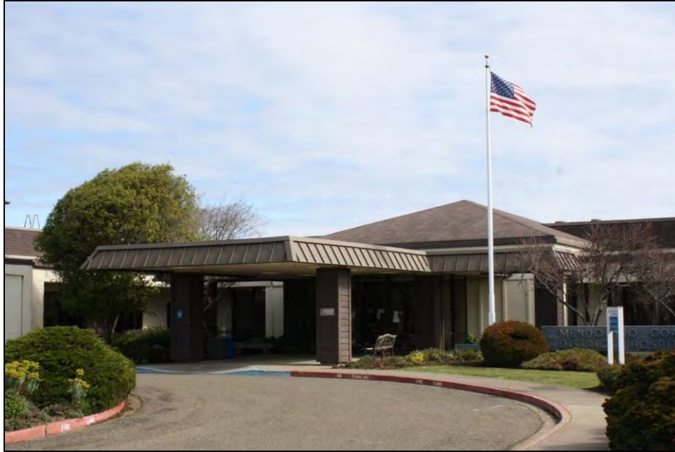
West (front) façade and front entry drive
