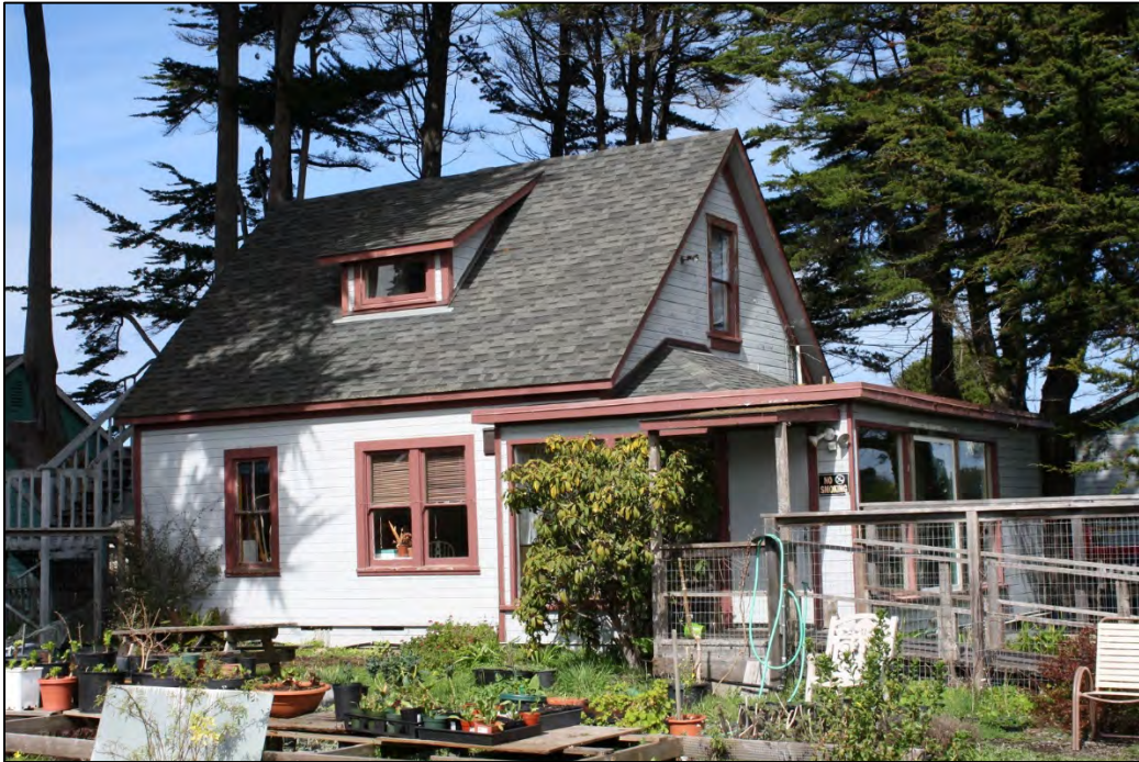
Rear (south) and east side façade, looking northwest
