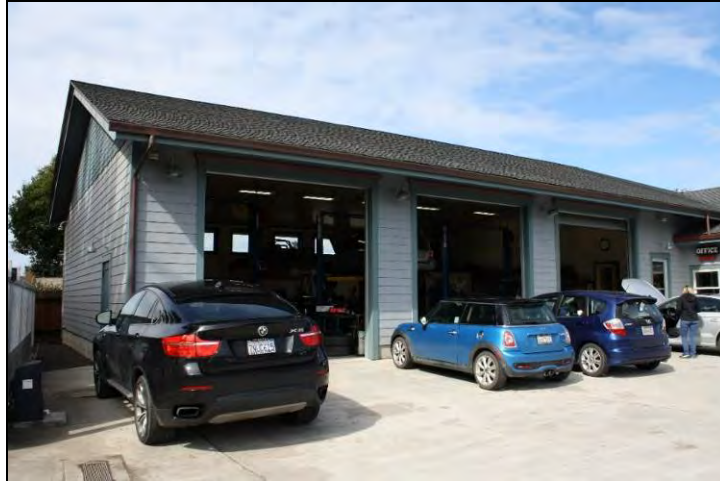
East (front) façade, south wing
