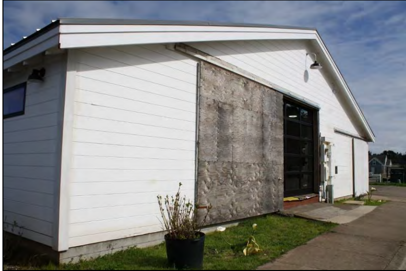
South (front) façade
