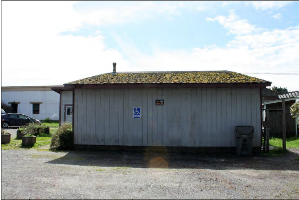
North side façade, looking south
