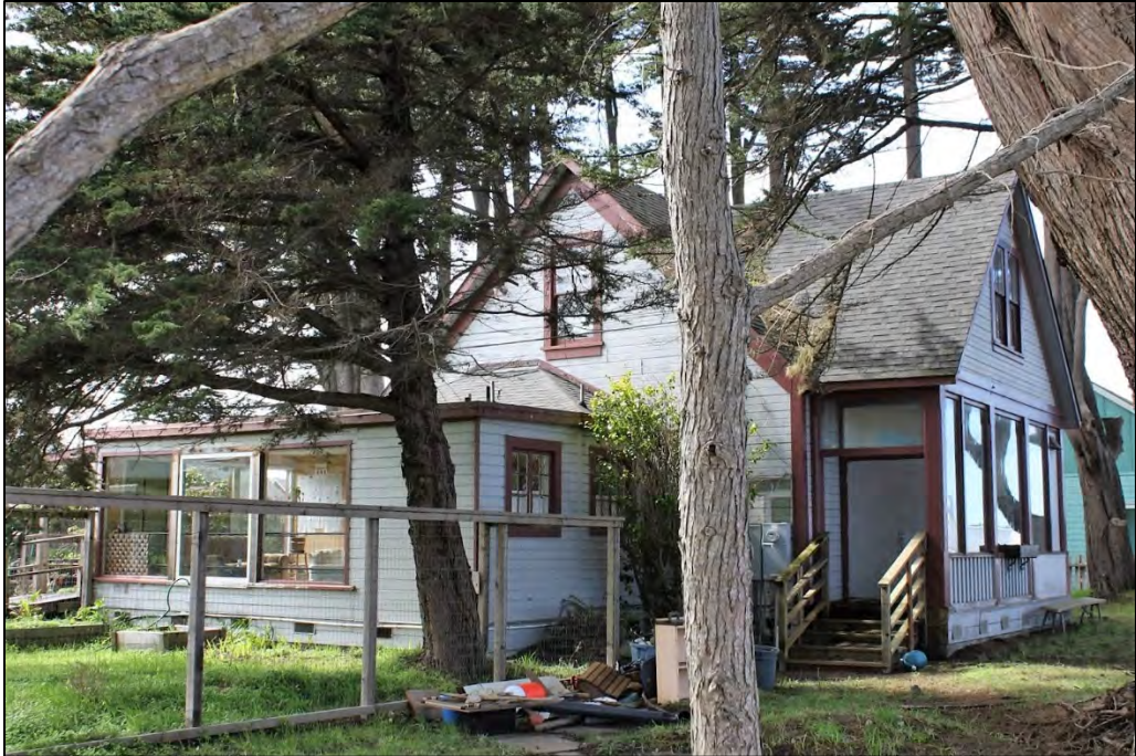
East side and front (north) façade, looking southwest
