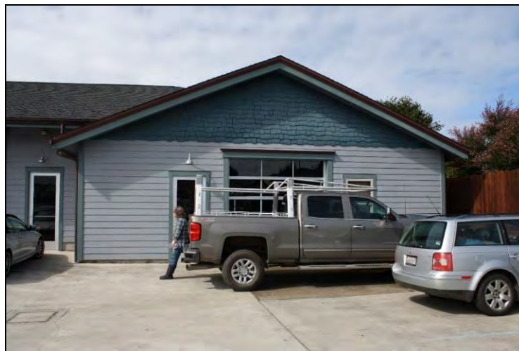
East (front) façade, north wing
