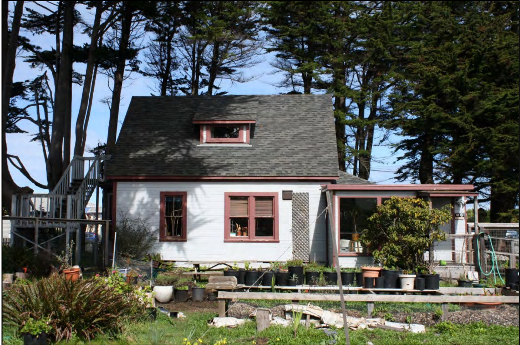
Rear (south) façade, looking north
