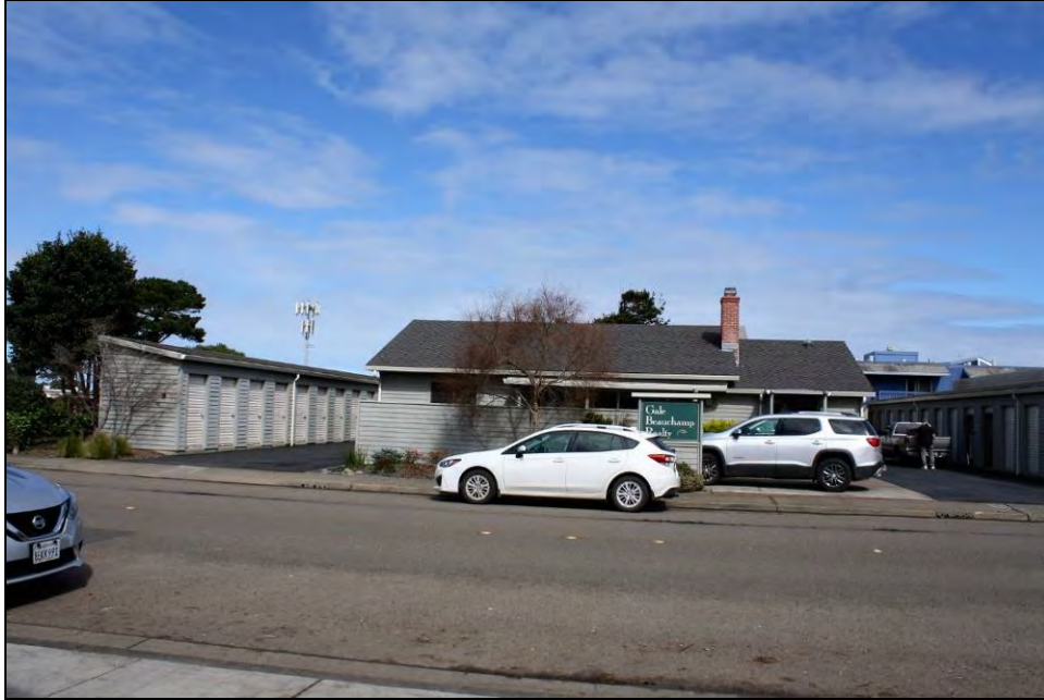
South (front) and east facades
