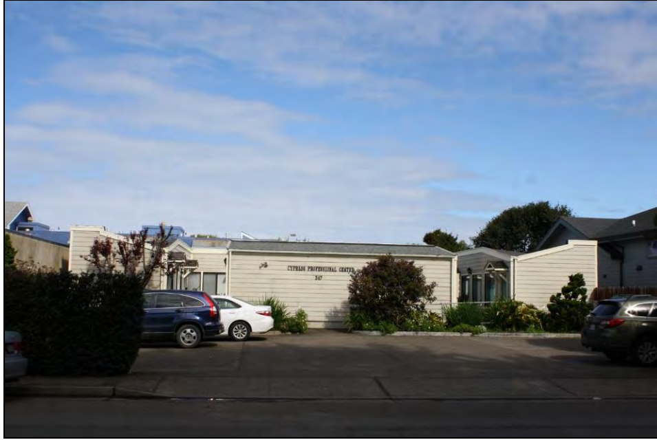
South (front) facade
