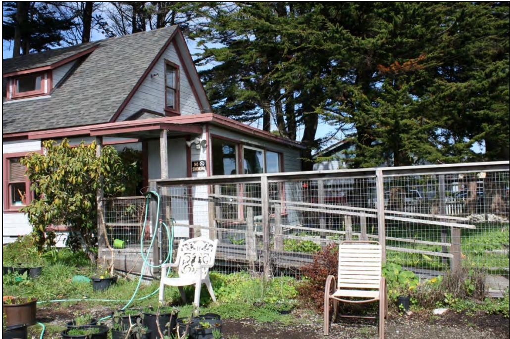
Handicap ramp and fences at southeast corner of house
