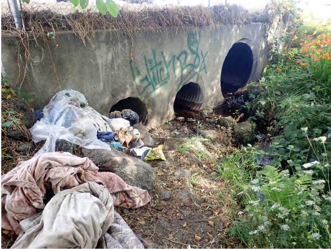
Figure 31. Culverts draining water onto the subject parcel from beneath Main Street.
