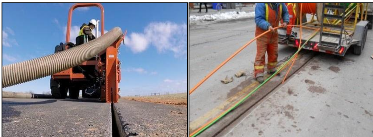
Figure 1. Micro-trenching
