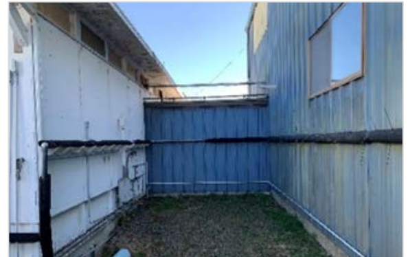
Blower room likely to be between buildings
