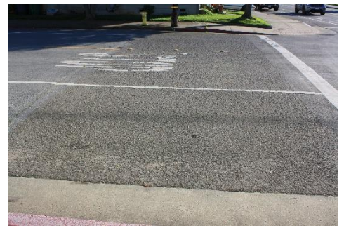
S. Franklin St. at Madrone St. - Change in pavement surface can be clearly seen on Madrone St. This project may consider extension of surface treatment limits to this location and other similar locations to present a continuous finished product.
