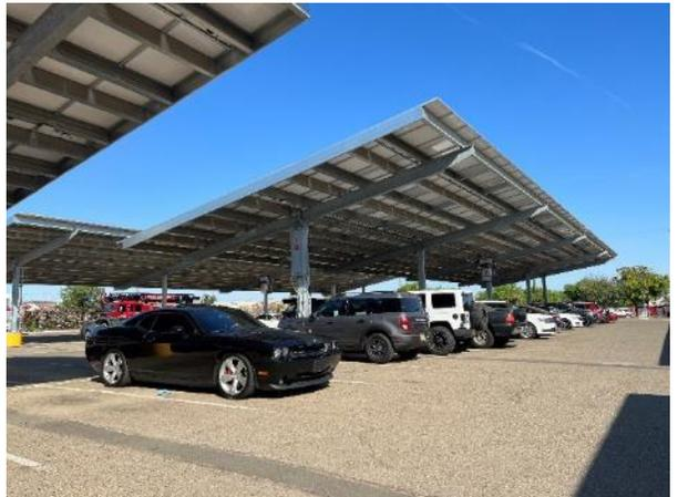
lot to the electrical grid is complicated, solar canopies over parking can directly provide electric current to on-site battery systems and electric vehicle charging.
