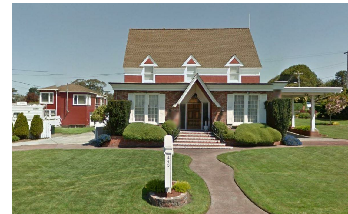
SITE PHOTO - SOUTH
