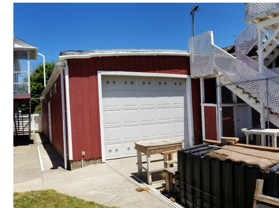
SITE PHOTO - GARAGE SOUTH
