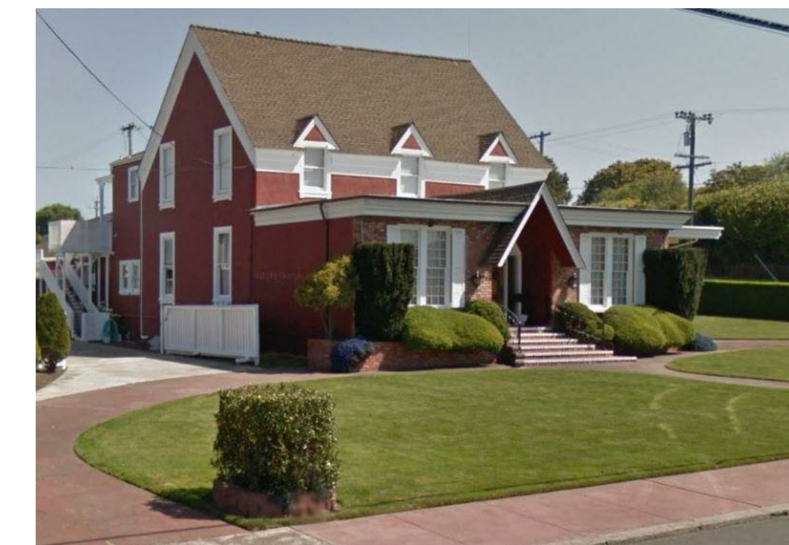
SITE PHOTO - WEST
