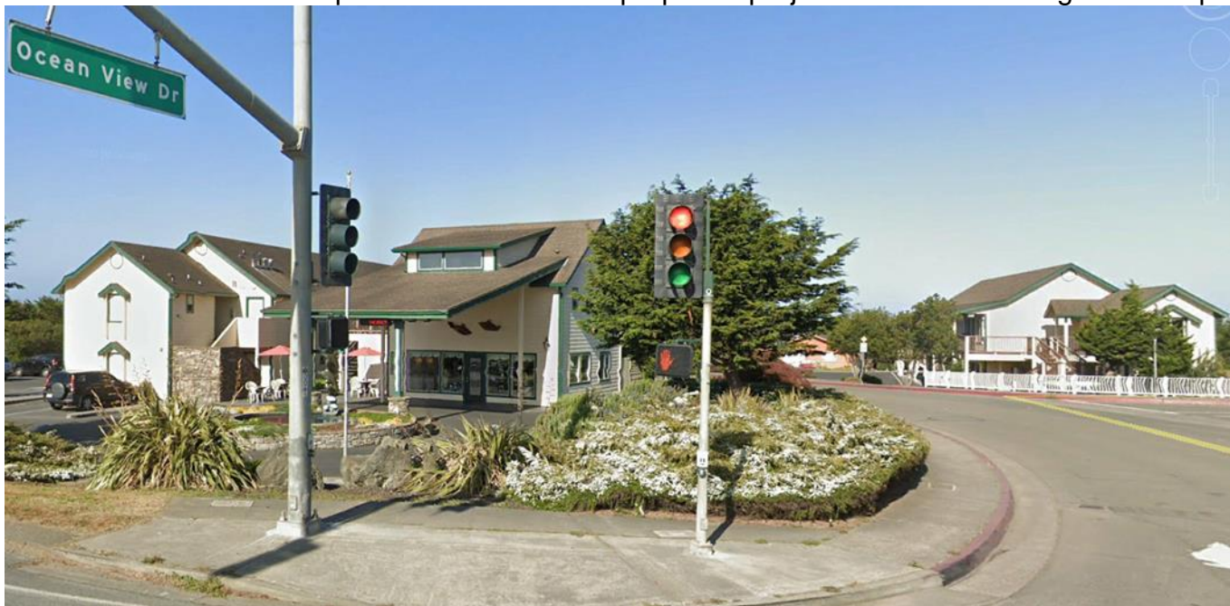
Image 1: Emerald Dolphin Motel Building A (right), Building B (left)
