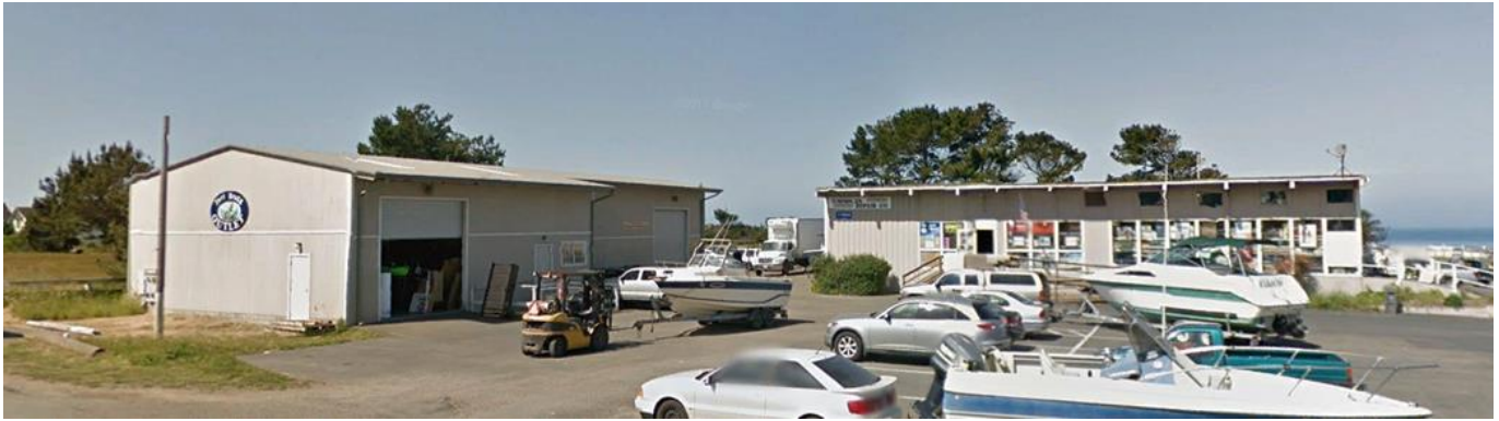
Image 2 : Fort Bragg Outlet Building A (right) and Building B (left)
